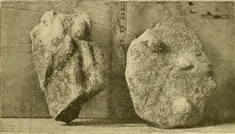
FIG. 2.—Iolite schist, showing projecting nodules.
