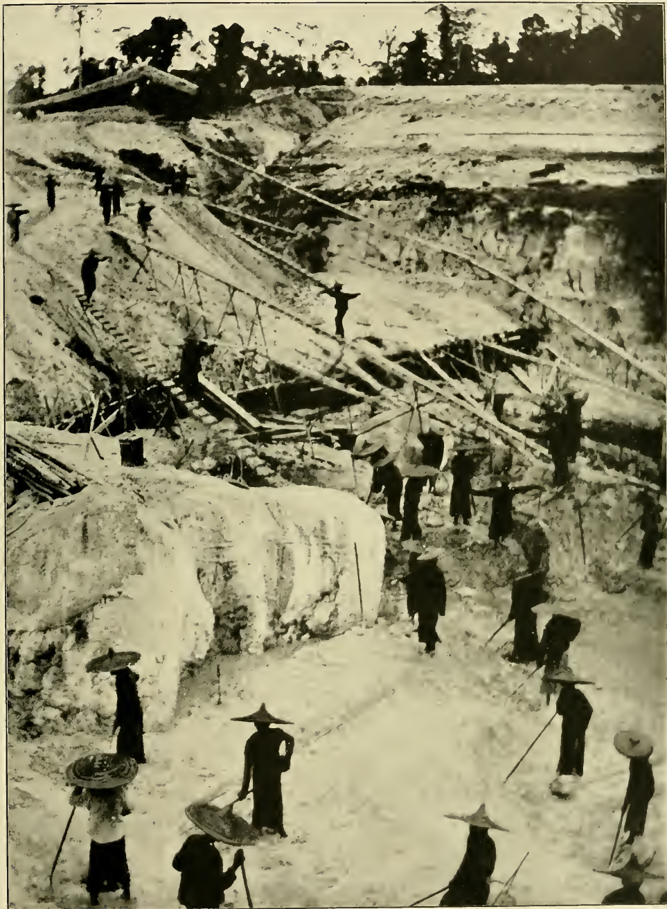
Tin mine near Tronoh, Perak, Malay peninsula, showing limestone bed rock underlying tin-bearing alluvium.
