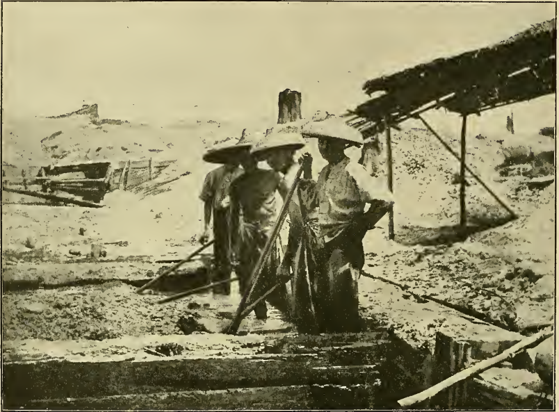
FIG. 8.—Washing tin ore near Tronoh, Perak, Malay peninsula.
