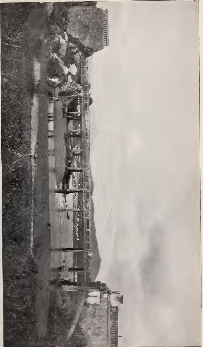
PIERS REMAINING OF FINE MASONRY BRIDGE ON MILITARY ROAD WASHED AWAY BY FLOODS.
