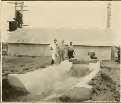
Electric pumps lift water from deep wells and from the San Joaquin river. Power costs about one cent or less per K. W. hour.
