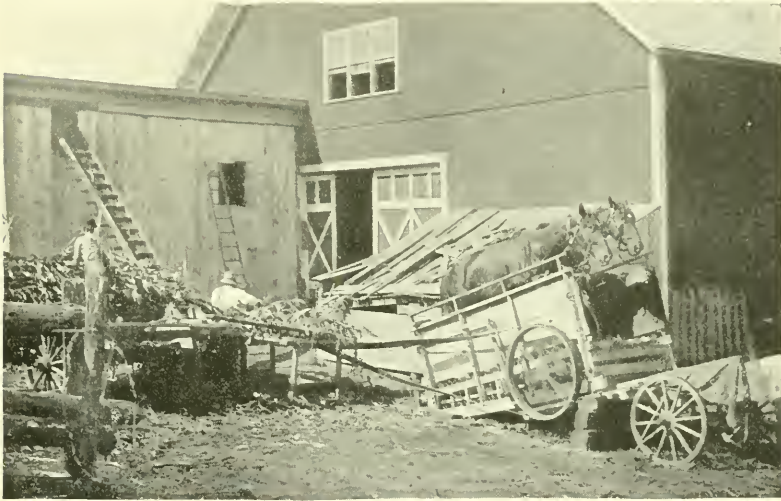
FILLING THE SILO
