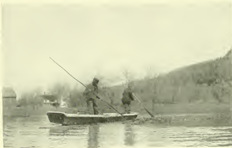
AFTER FLOOD TRASH
