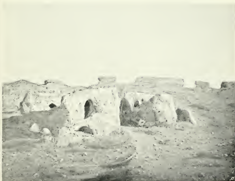
PRESUMED SUMMITS OF TOWERS BURIED IN SAND, ZAIDAN. Notice top of Castellated Wall behind.
