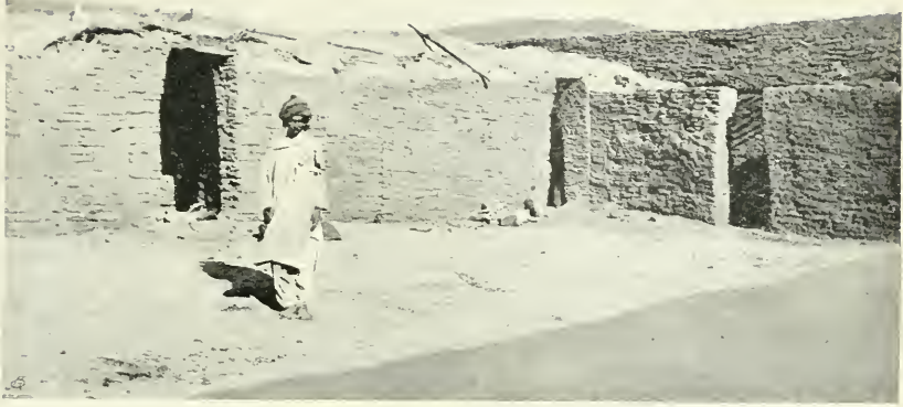
INTERIOR OF REST HOUSE, MUKAK.
