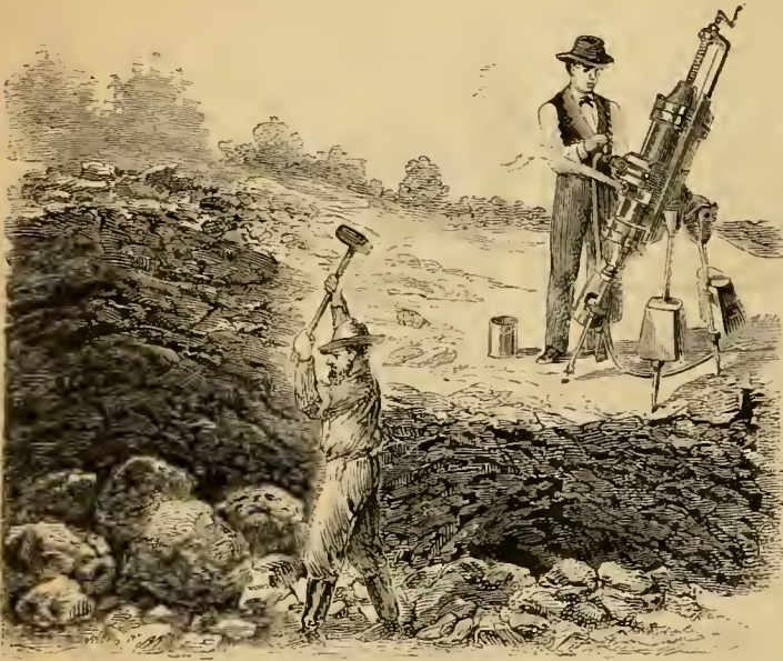
Fig. 1.—WARING'S ROCK-DRILL.
