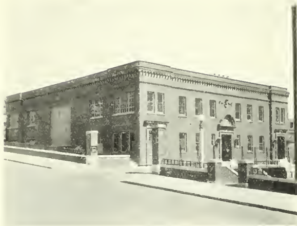
View of Pathological Building
