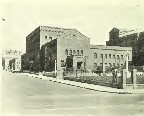
View of Receiving Building and Emergency Hospital
