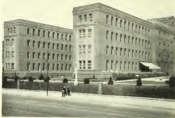
Typical Ward Building
