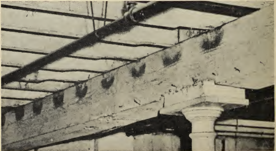
Fig. 5. Smears made by rats traveling along a supporting floor beam. The rats must crawl along the side of the beam under each joist, and thus leave the U U U U-shaped markings. Courtesy of U. S. Public Health Service.
