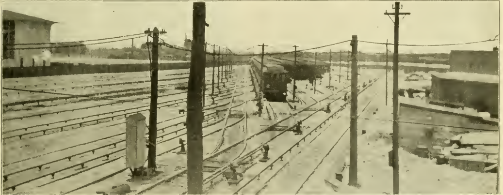
South Side Elevated Railroad—Sixty-third Street Storage Yards.
