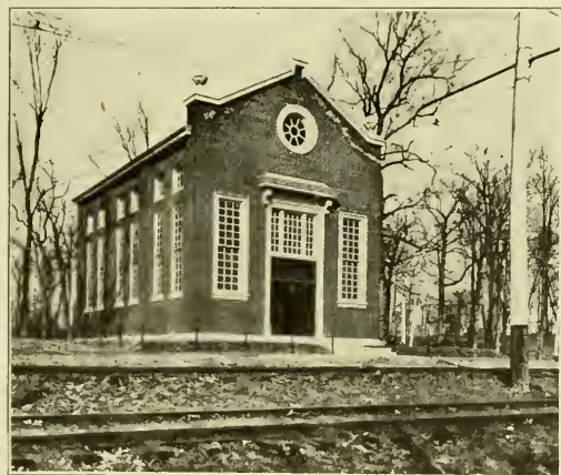
United Railways of St. Louis—Creve Coeur Substation.
