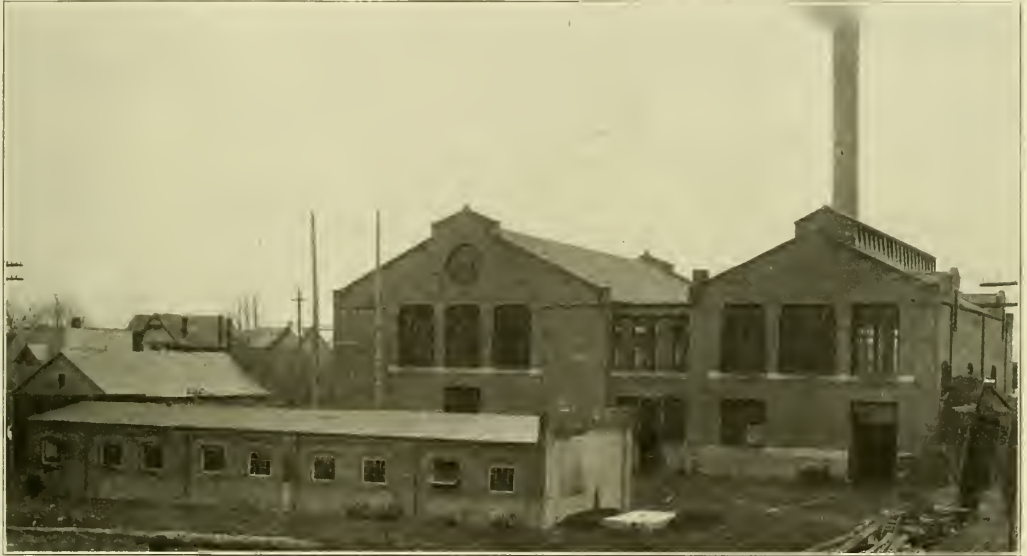
Kokomo Marion & Western—General View of Power Plant, with Storage Battery House in Foreground.
