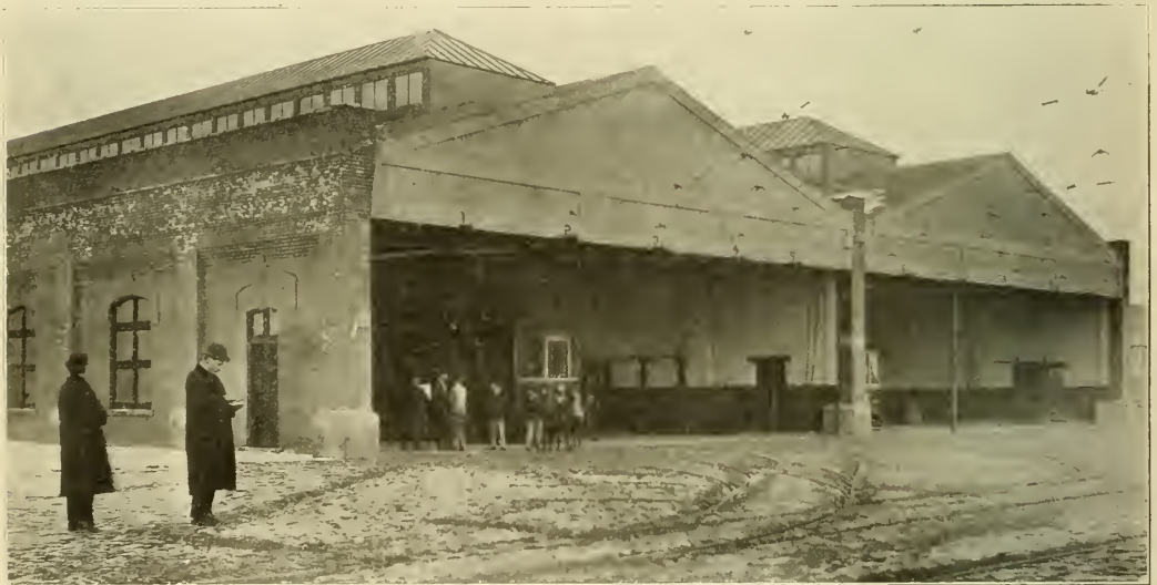
Broadway Car House, Buffalo—Front End of Car House.
