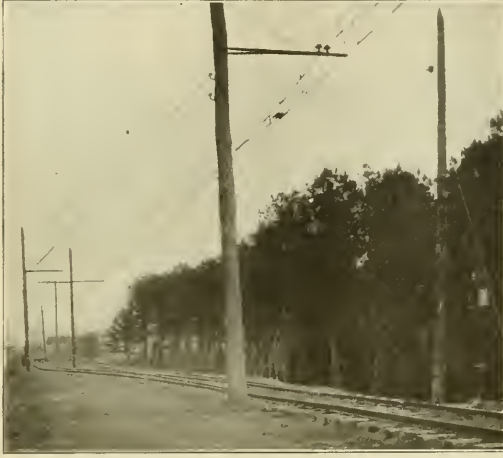
Richmond & Chesapeake Bay Railway—Catenary Construction at Turnout.
