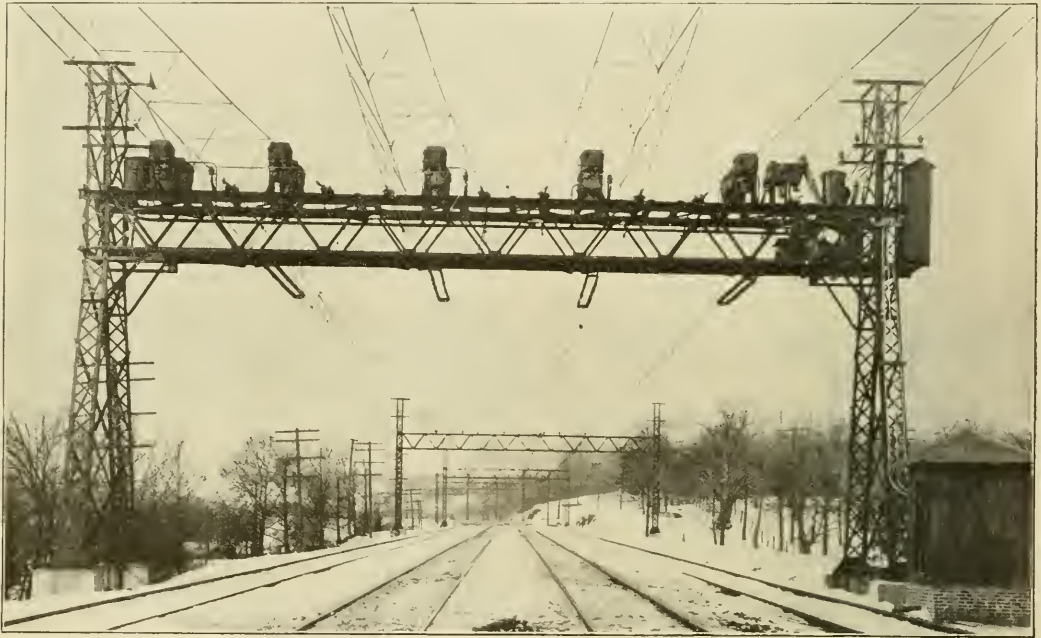
New York New Haven & Hartford Single-Phase System—Anchor Bridge and Catenary Construction.
