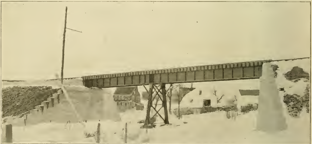
Hanover & York Railway—Overhead Crossing with Highway and Stream.
