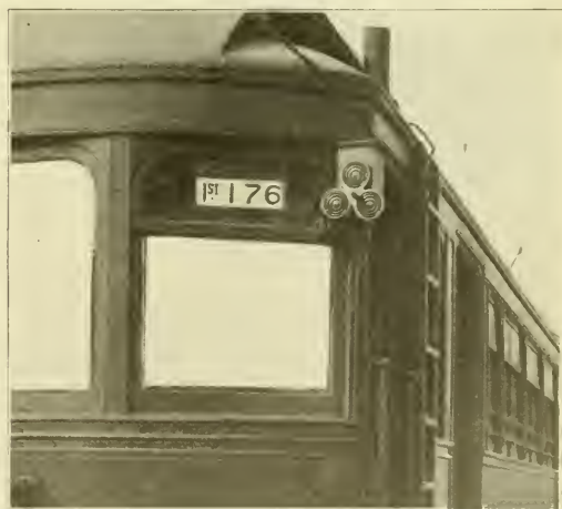
Gibbs Train-Indicating Device—View as Installed in Car.
