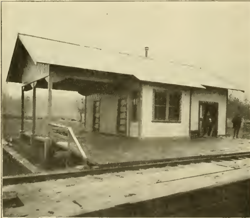
Oregon Electric Railway—Standard Local Passenger Station.
