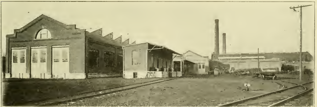
Anderson Shops Indiana Union Traction Company—South End, Exterior.
