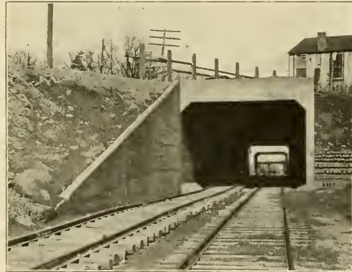
Washington Baltimore & Annapolis—Concrete Subway at Baltimore Entrance.
