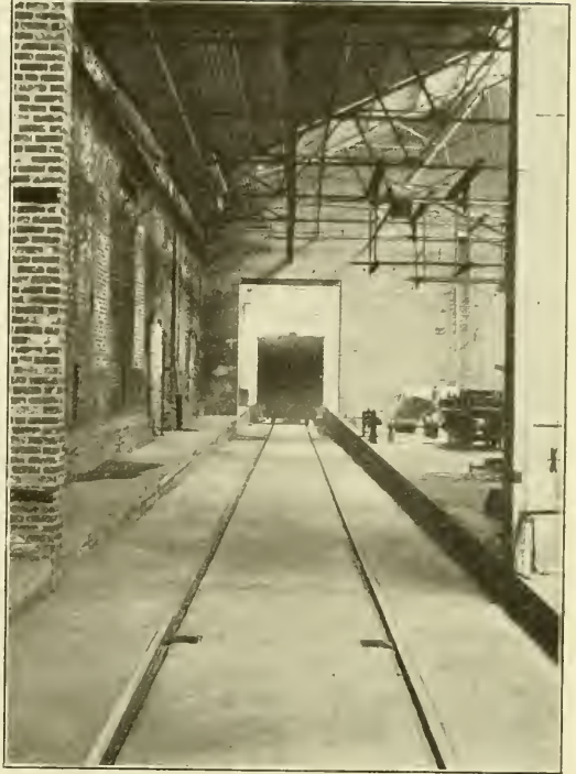
Anderson Shops Indiana Union Traction Company—Depressed Track Through Storeroom.
