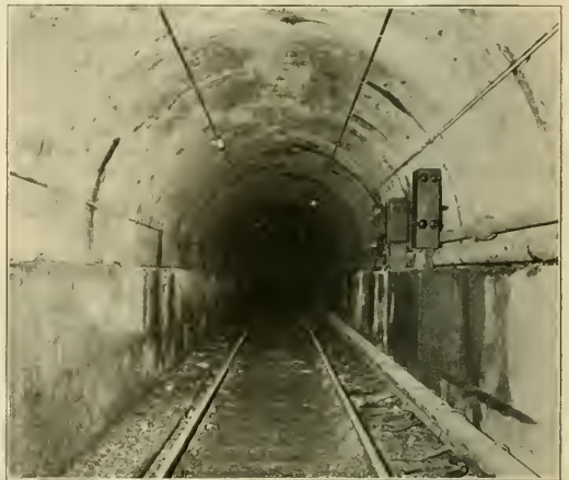
Hudson River Tunnel—First Signal Station.
