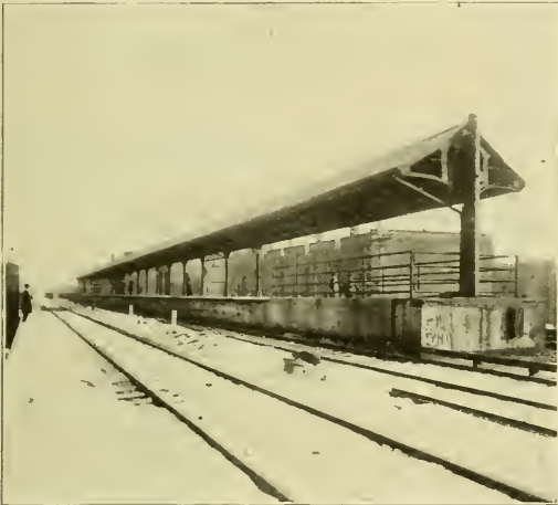
South Side Elevated Railroad—Long Station Platform on Kenwood Extension.
