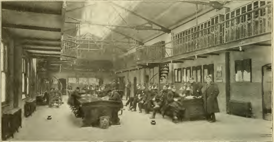
Broadway Car House, Buffalo—Trainmen's Quarters.
