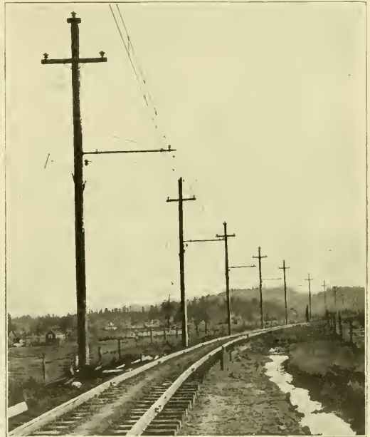
Oregon Electric Railway—Transmission Bracket and Catenary Construction on Curve.
