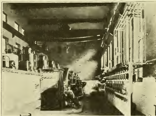
United Railways of St. Louis—Spring Avenue Substation.
