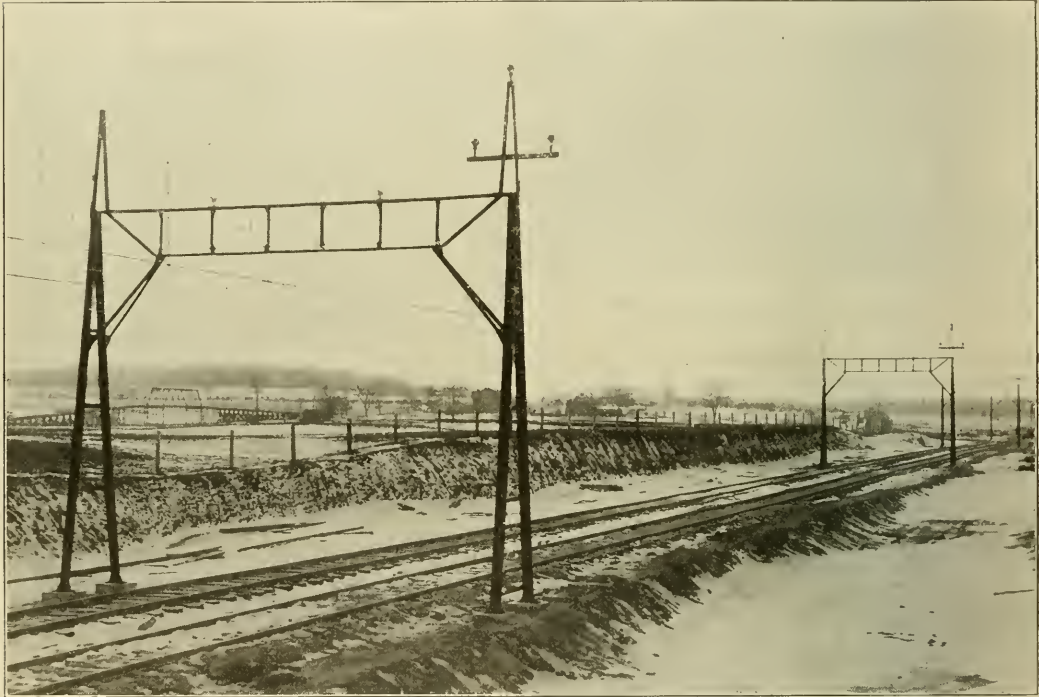
Syracuse Lake Shore & Northern Railroad—Catenary Trolley Construction and Power Transmission Line.
