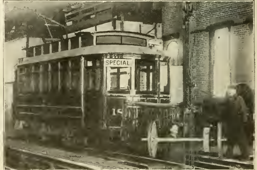
Allegheny Shop Practice—View of Wheels Being Raised from Repair Pit.
