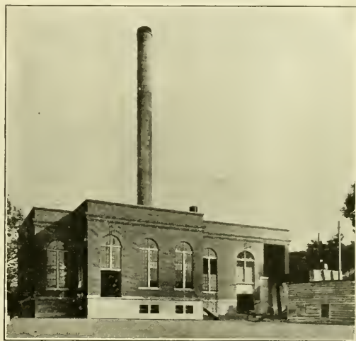
Ben-Hur Route—Power Station Building.
