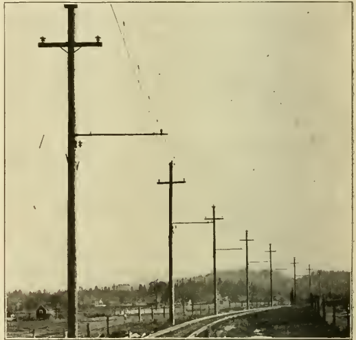
Oregon Electric Railway—Overhead Construction on Curve.
