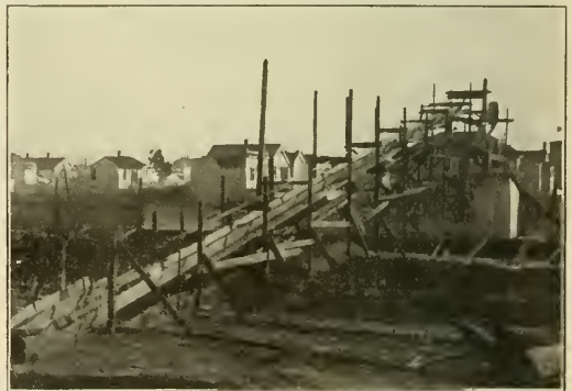
Key Route Power Station—A Simple Conveyor for Removing Dirt.
