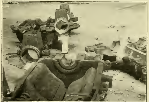
Indiana Union Traction—Group of Thermit Welds.
