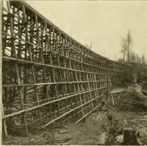
Oregon Electric Railway—Long Timber Trestle on Curve Near Portland, 100 Feet High.
