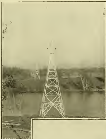
Steel Tower Construction for Long Spans
