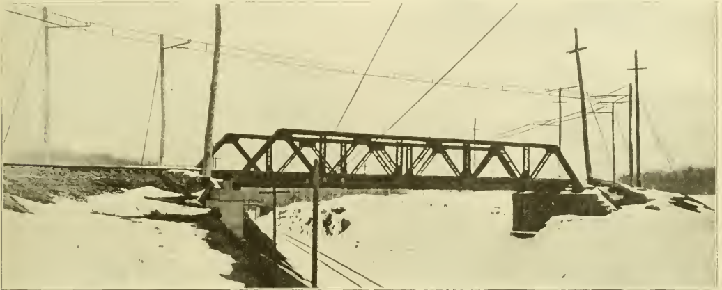
Hanover & York Railway—Overhead Crossing with Steam Railway.
