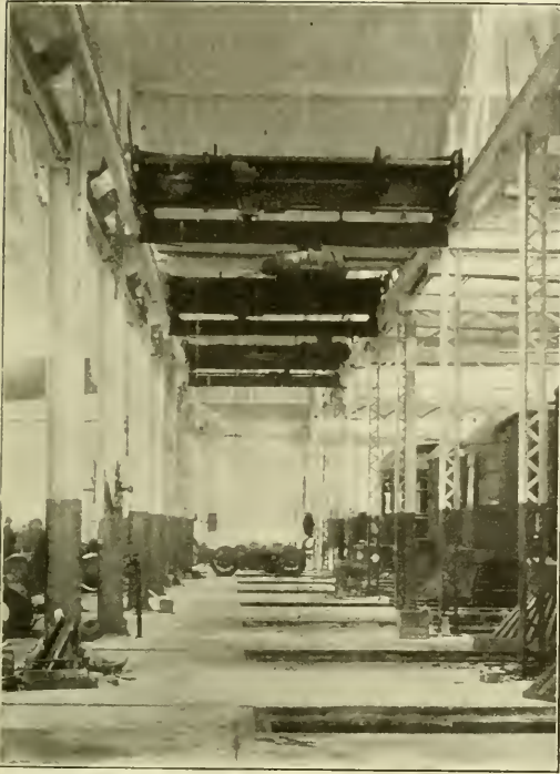
Anderson Shops Indiana Union Traction Company—Truck Aisle with Traveling Cranes.
