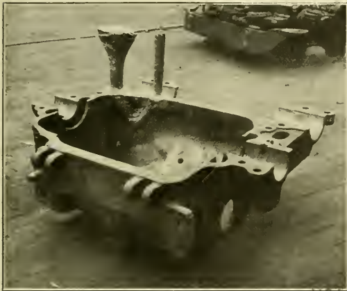
Chicago City Railway—Motor Shell with Thermit Repair.
