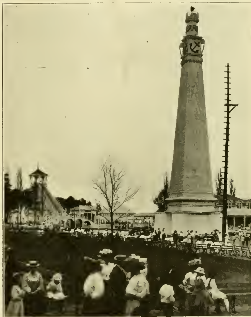
Scarboro Beach Park, Toronto—Electric Tower and Chutes.
