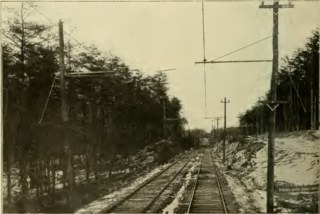
Washington Baltimore & Annapolis—Overhead Construction on Main Line.
