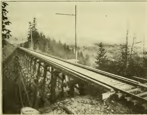
Oregon Electric Railway—Long Timber Trestle Near Portland.
