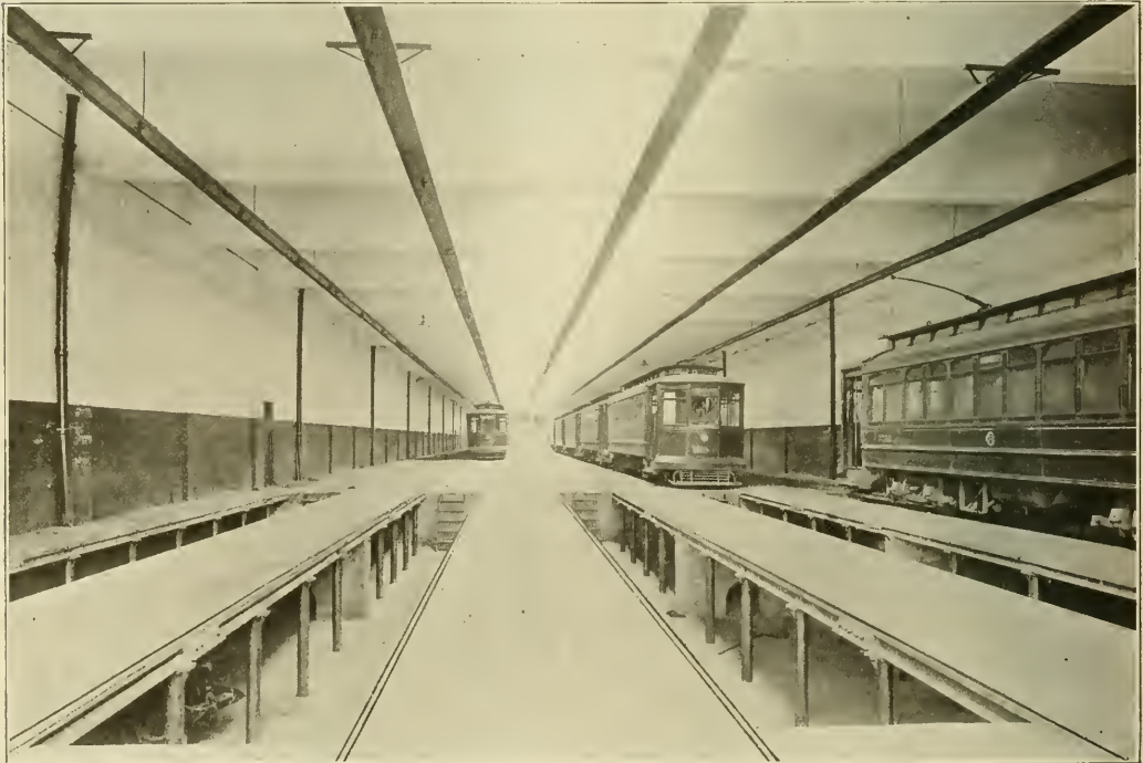
Chicago City Railway—Interior View of One Bay in New Car House.
