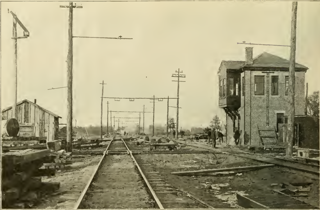
Washington Baltimore & Annapolis—Interlocking Tower at Naval Academy Junction.
