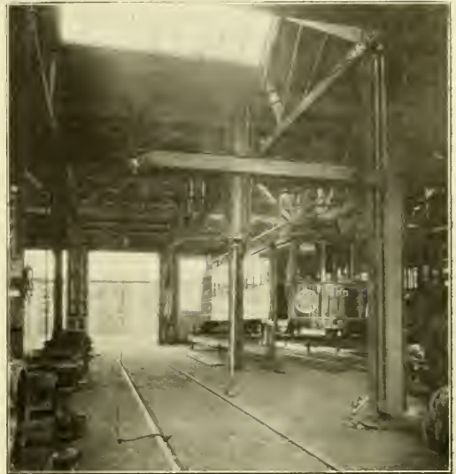
Emeryville Shops—View of Crane as Installed.
