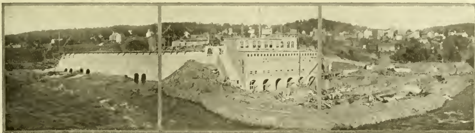
Taylor's Falls Power House and Dam.
