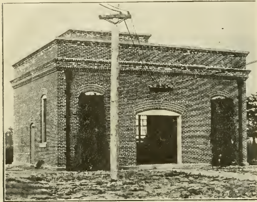
Ben-Hur Route—Substation Building.
