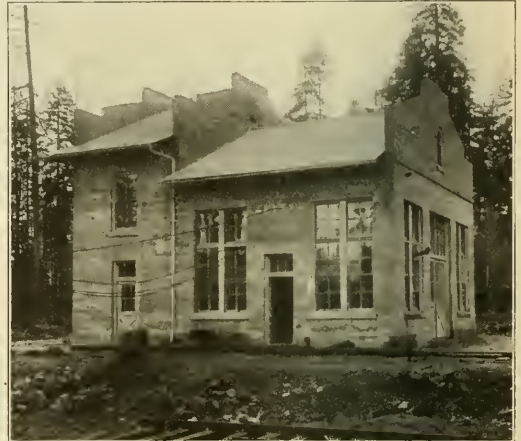
Oregon Electric Railway—Standard Concrete Substation.
