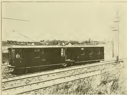
United Railways of St. Louis.—Portable Substation in Two Cars.
