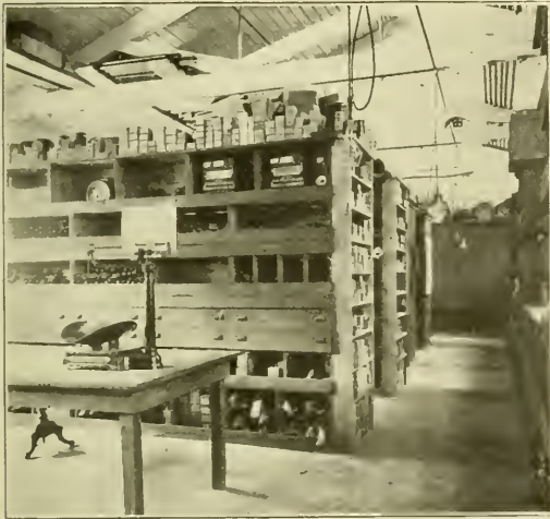
York Shops—Stock Racks in Storeroom.
