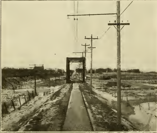
Chicago & Southern—Typical Roadway, Bridge and Overhead Construction.
