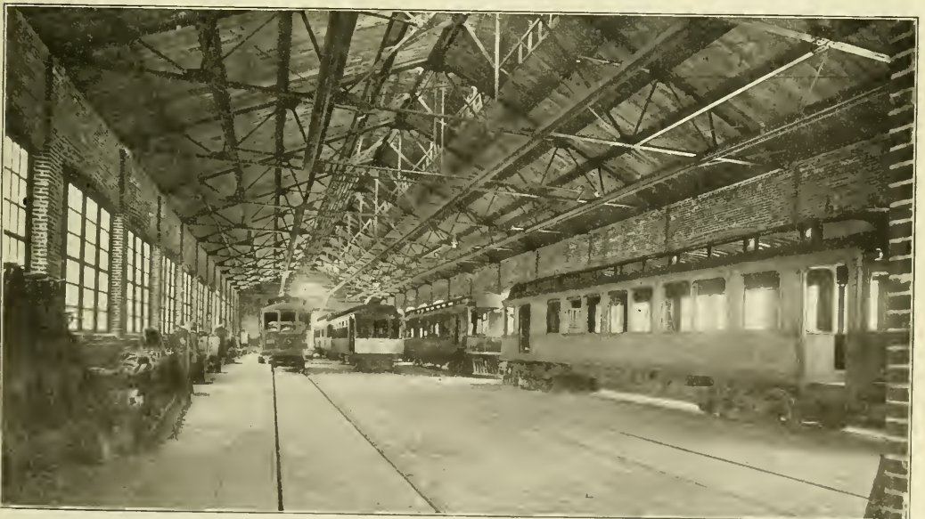
Anderson Shops Indiana Union Traction Company—Paint Shop with Three Through Tracks, a Concrete Floor and a Generous Window Illumination.
