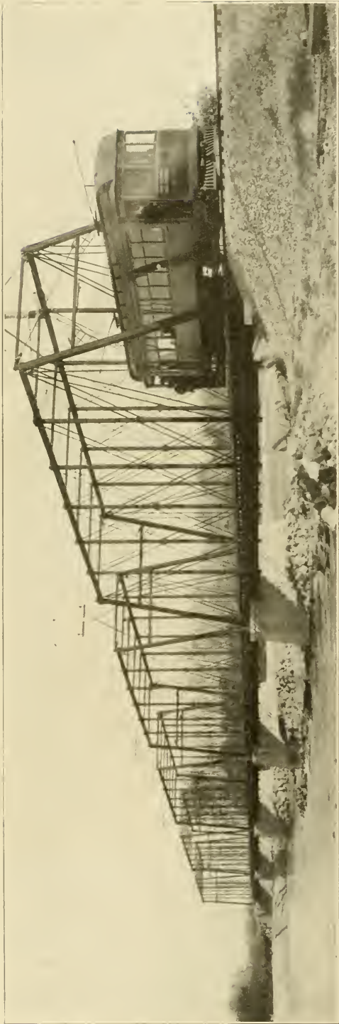
Boise & Interurban Railway—Steel Truss Bridge, 550 Feet Long, over Boise River, Showing Interurban Passenger Car.
