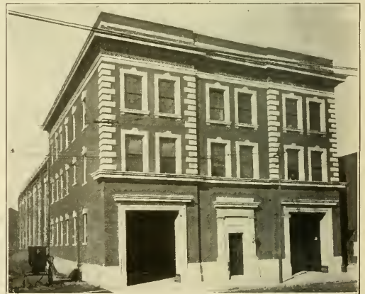
United Railways of St. Louis—Spring Avenue Substation and Emergency Station.
