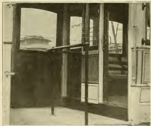
Cleveland Pay-As-You-Enter Car—Showing Arrangement of Rear Platform.
