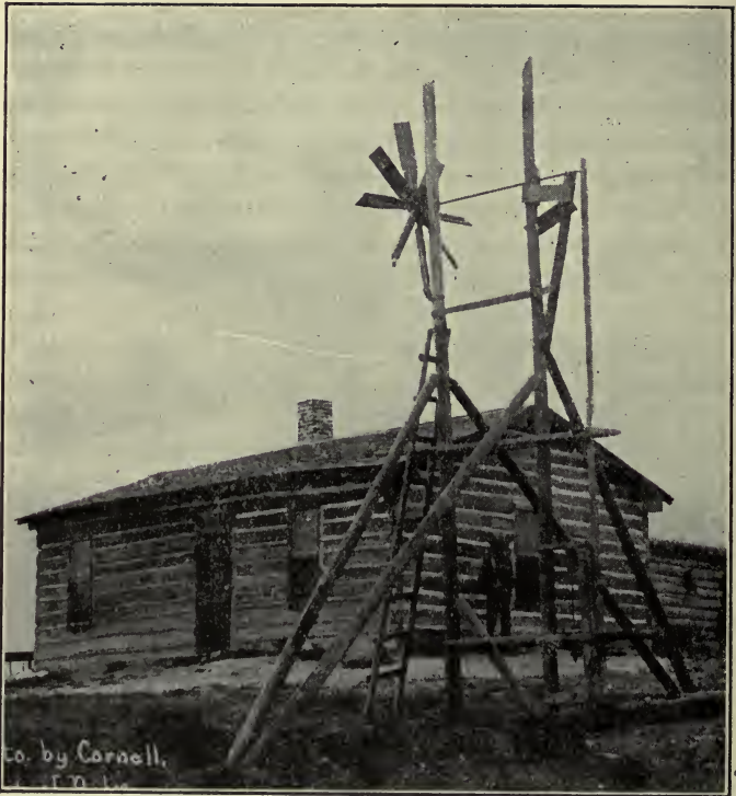
FIG. 204—MOCK TURBINE WINDMILL
