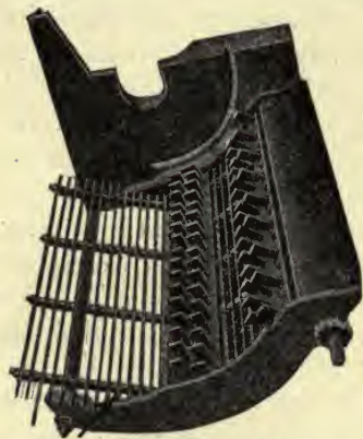
FIG. 158—THE GRATE AND CONCAVE
