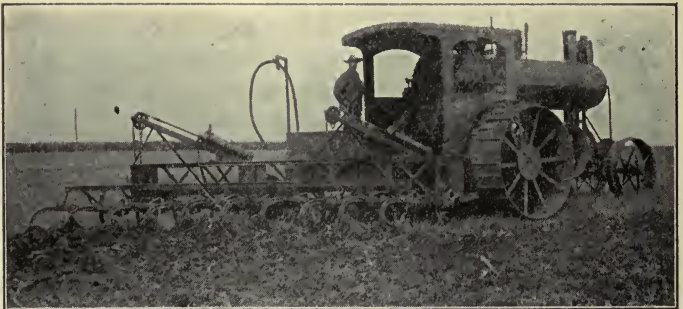
FIG. 329—LOCOMOTIVE TYPE OF TRACTION ENGINE WITH STEAM-OPERATED PLOW
