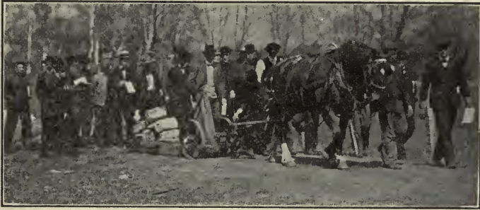
FIG. 197—OBTAINING THE WORK OF A HORSE WITH A RECORDING DYNAMOMETER
