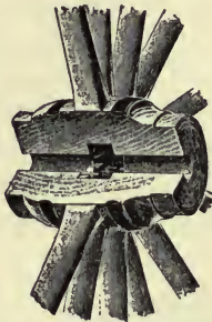
FIG. 186—A COMPRESSED WHEEL HUB
