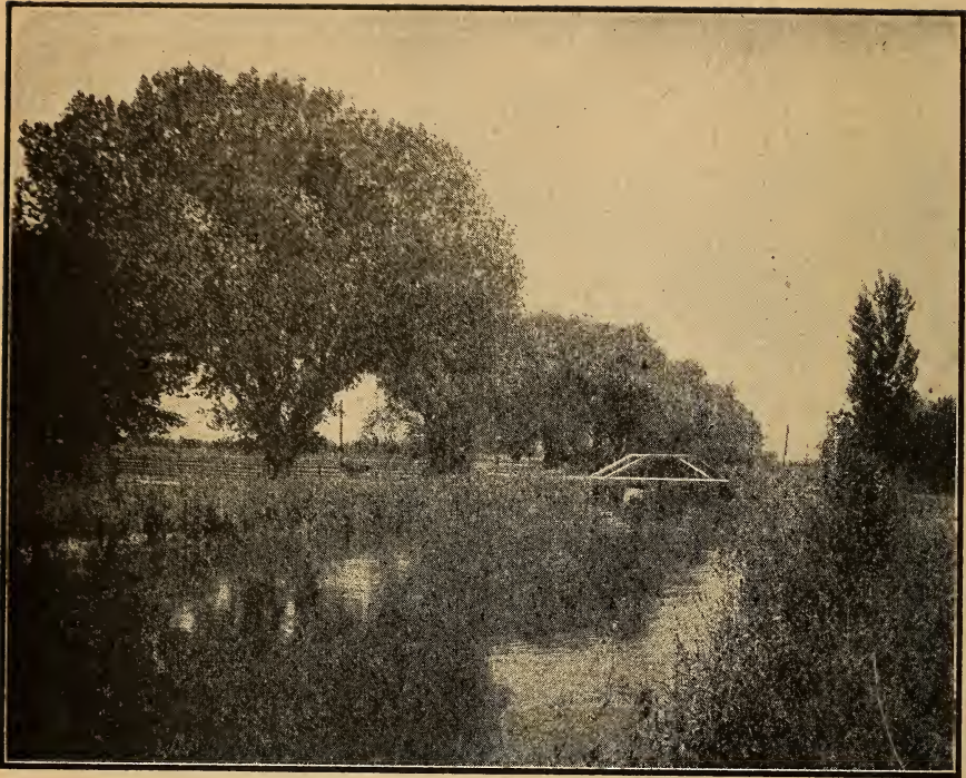
Fresno Irrigating Canal
