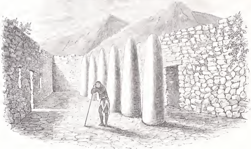
GRAND HALL OF THE MAIN BUILDING OF THE SECOND GROUP.
