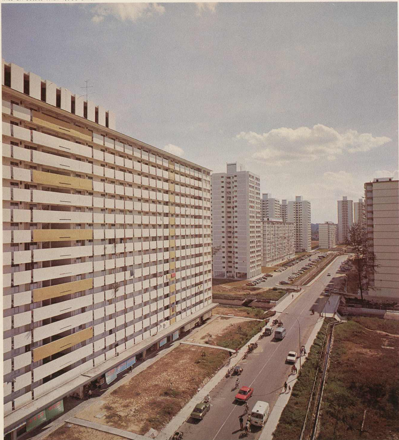
Balestier Estate Redevelopment where the single-storey artisan quarters built before the war were demolished for redevelopment into an estate with 4,900 units.
