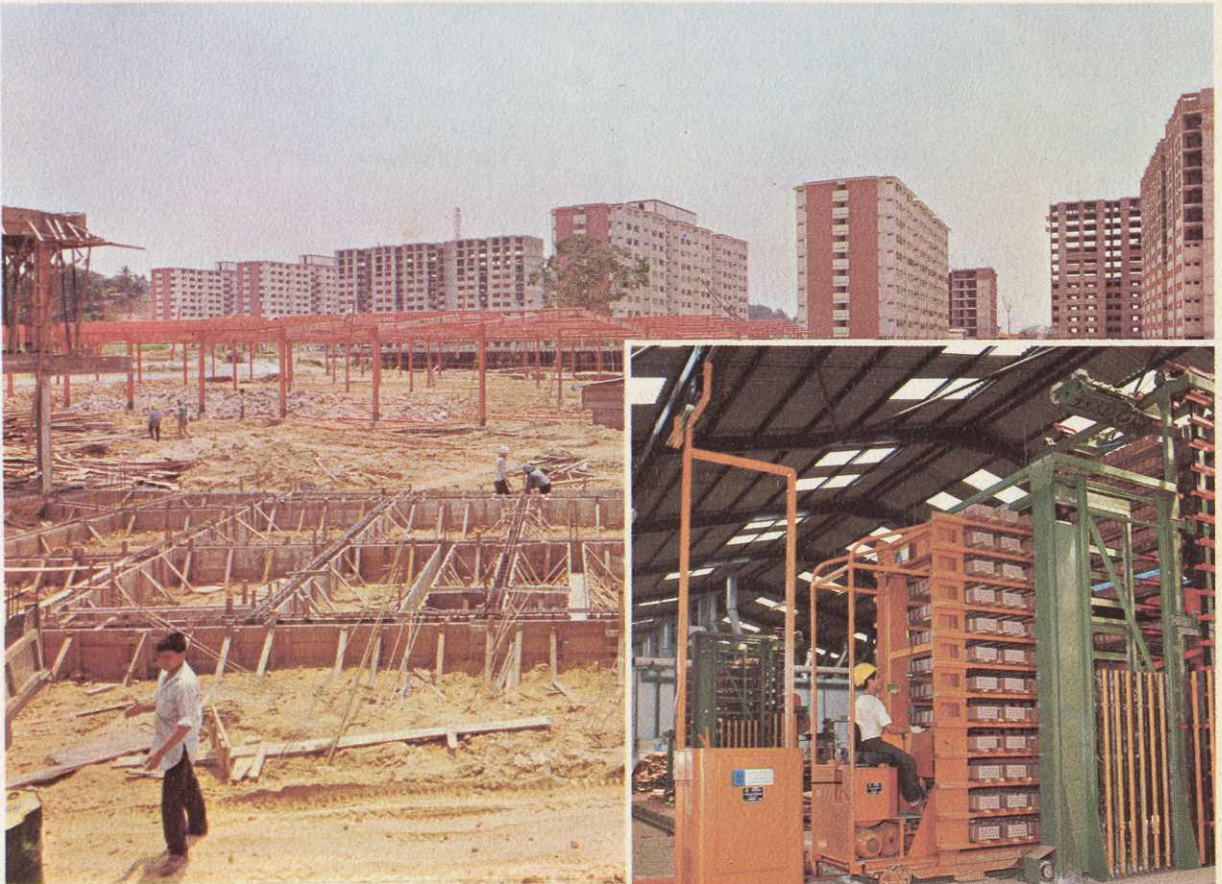
The Board's flats under construction in Kampong Chai Chee.
