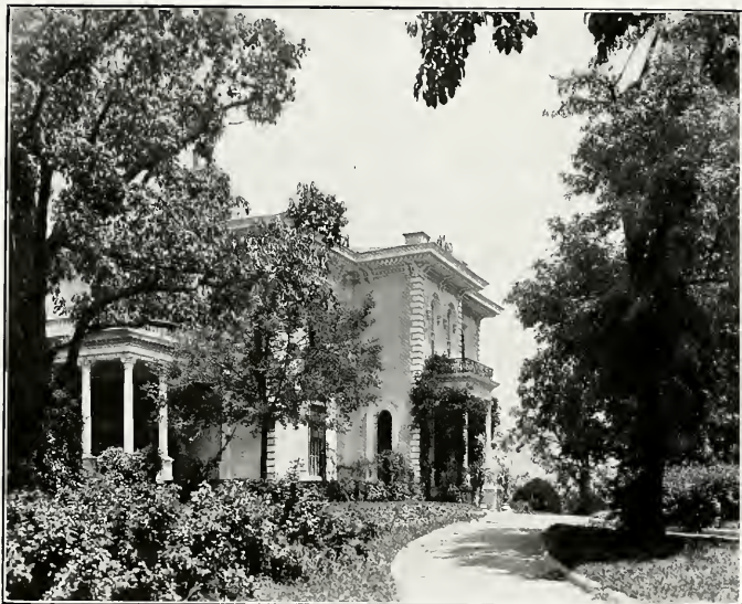
WARD PLACE—APPROACH FROM SOUTHWEST
