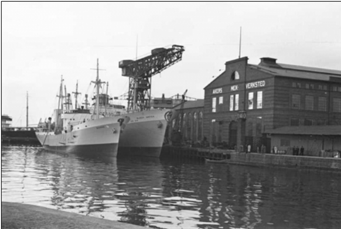
Figure 15. Akers Mek Verksted: Shipyard in Oslo 164
