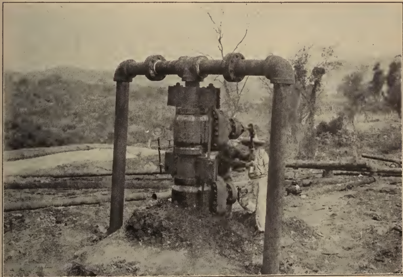
When this well came in it blew the drilling derrick sky high. Finally it was brought under control and it now flows its hundreds of barrels of oil through pipelines connecting it with a big tank at tidewater.
