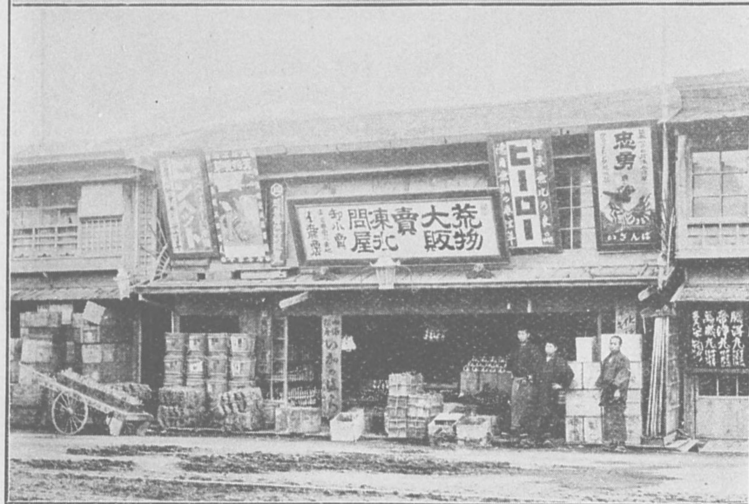
店貨雜榛近 ④ 町濱東港館函 KONDOW, Grocery, Higashi-hama-machi, Hakodate.
