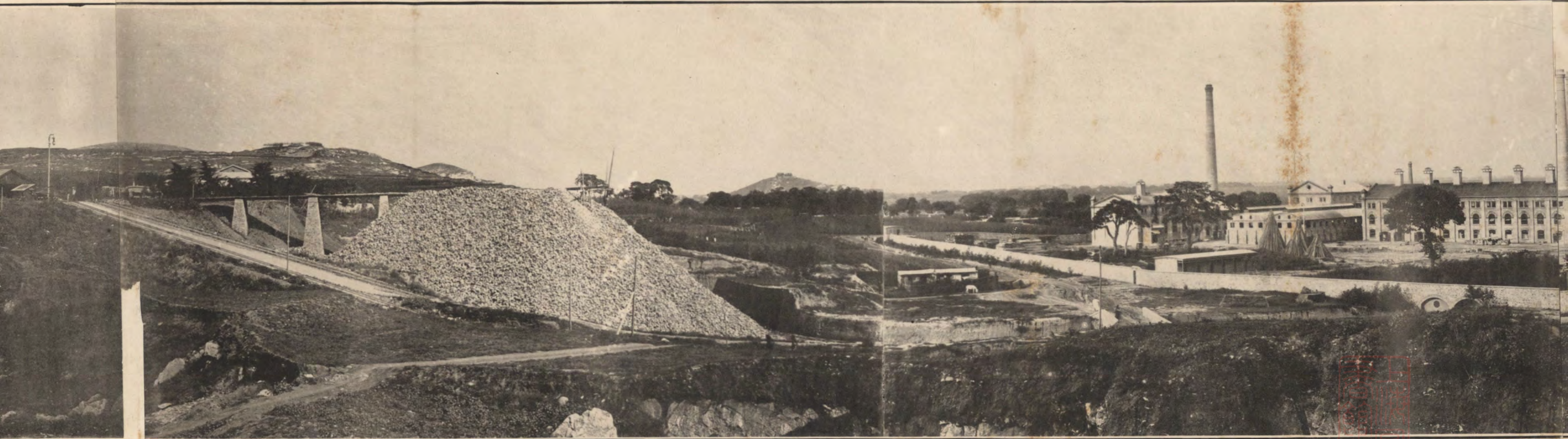
FULL VIEW OF THE CHEE HSIN CEMENT WORKS, TANGSHAN.
