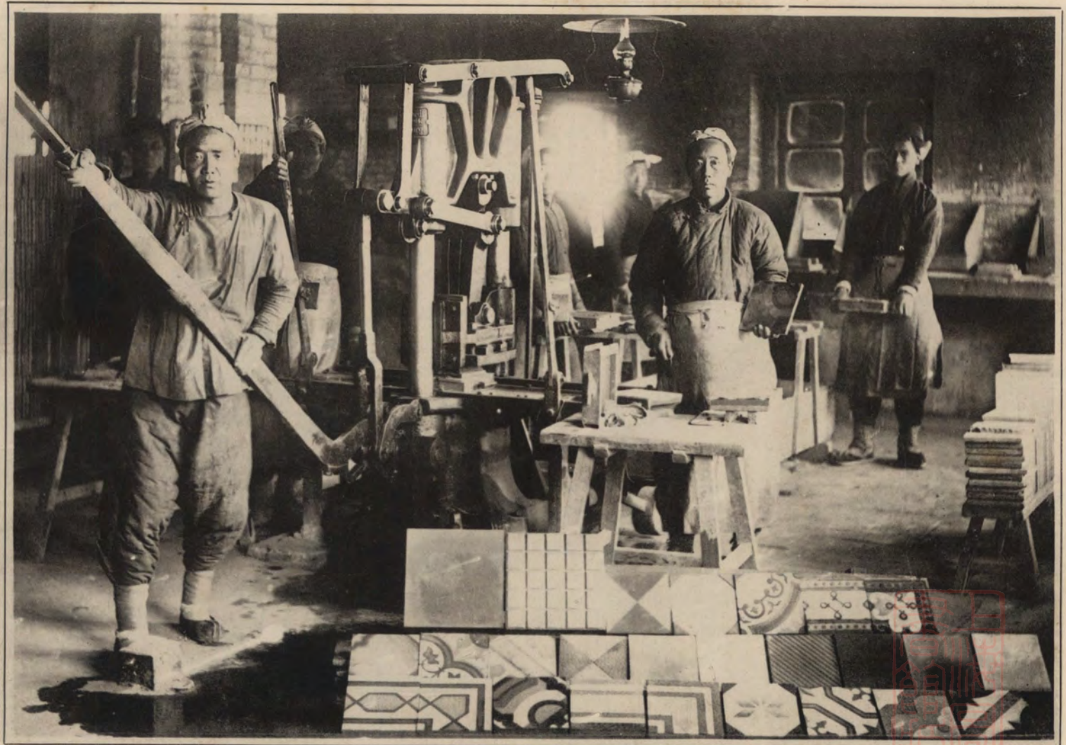
MOSAIC TILES MANUFACTORY.
