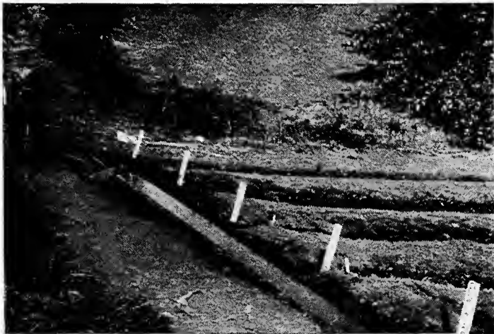
82. IRRIGATING A GARDEN FROM A HYDRANT IN A SEMI- ARID REGION (PULLMAN, WASH.)
