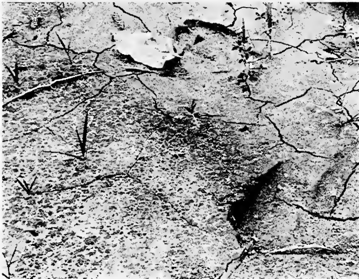
31. A CLAY SOIL CRACKING
