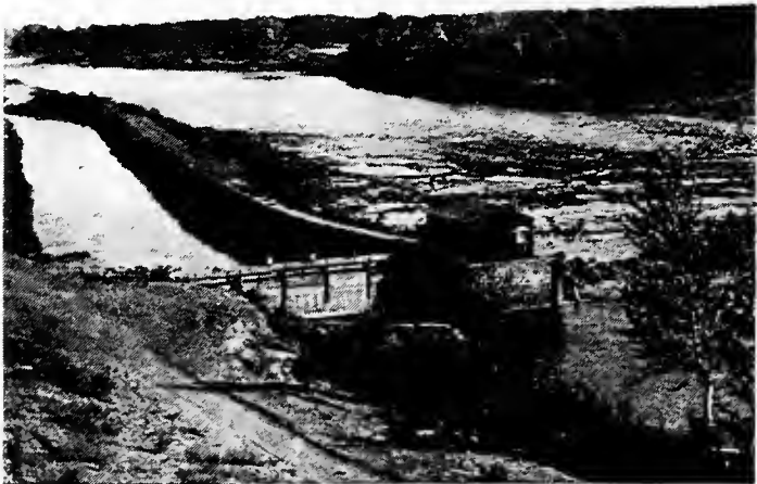
81. THE INTAKE OF THE SUNNYSIDE CANAL, YAKIMA VALLEY, WASHINGTON Note the head-gate. These large canals are usually built by corporations or partnerships of farmers
