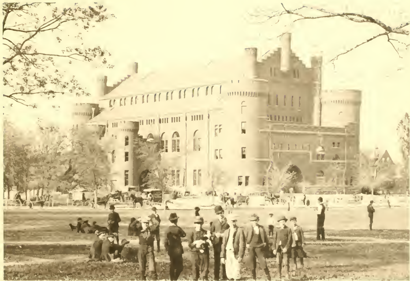
ARMORY AND GYMNASIUM.
