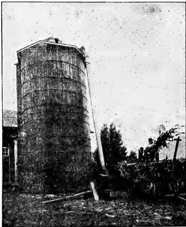
Fig 43—Filling Silo with Blower
