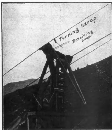
RUTTLE TURNING STRAP FOR TRAMWAY CABLES
