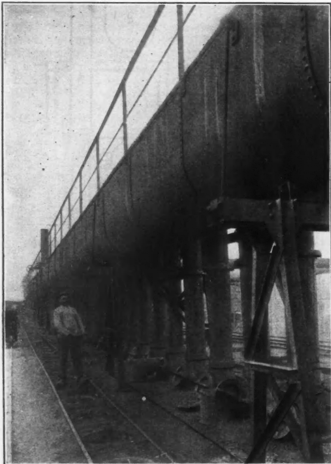
FIG. 2. SHOWING SCHEME FOR ELIMINATING THE FUMES EVOLVED BY THE CHARGING OF COKE OVENS
