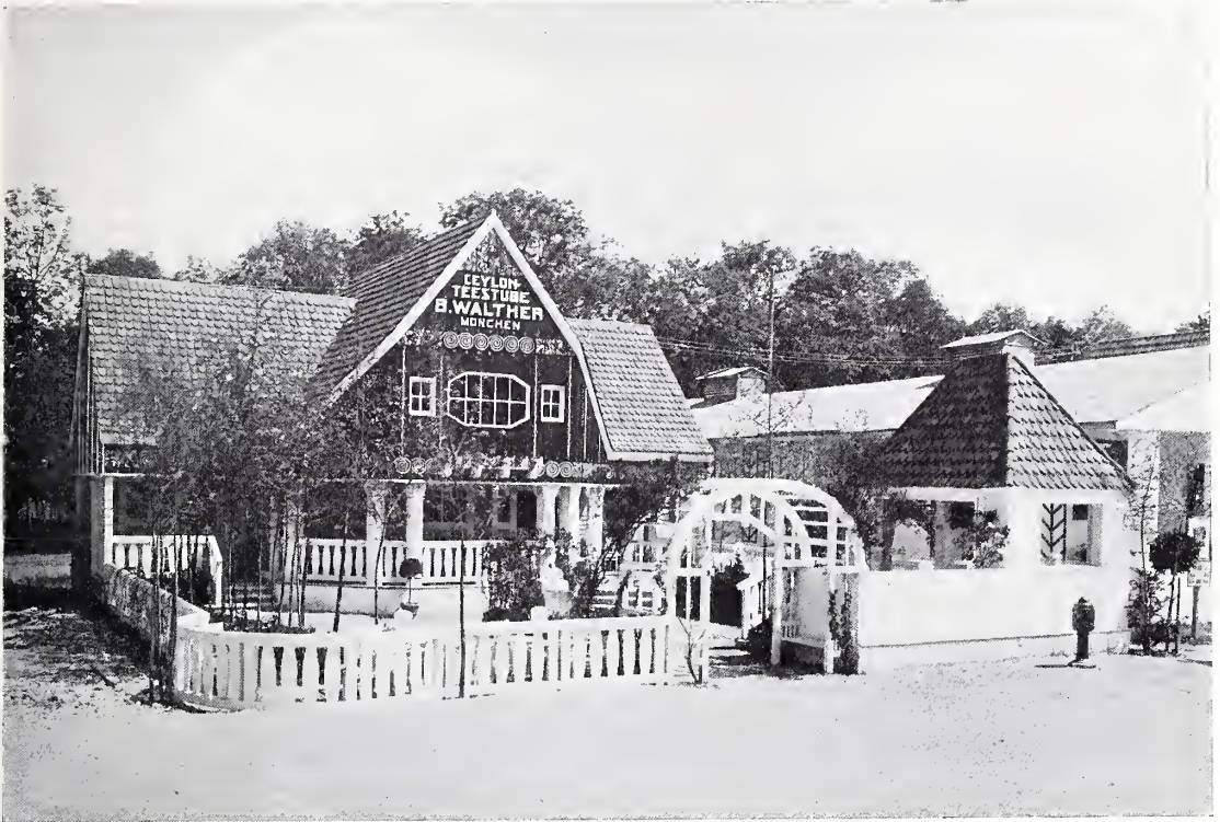
MUNICH EXHIBITION : TEA HOUSE IN THE RECREATION GROUND
