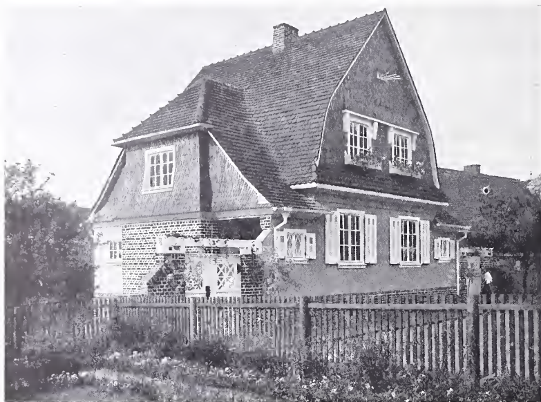
PAIR OF SEMI-DETACHED COTTAGES FOR ARTISANS DESIGNED BY MAHR & MARKWORT, ARCHITECTS, FOR DVCKERHOFF & SÖHNE OF AMÖNEBURG ON RHINE
