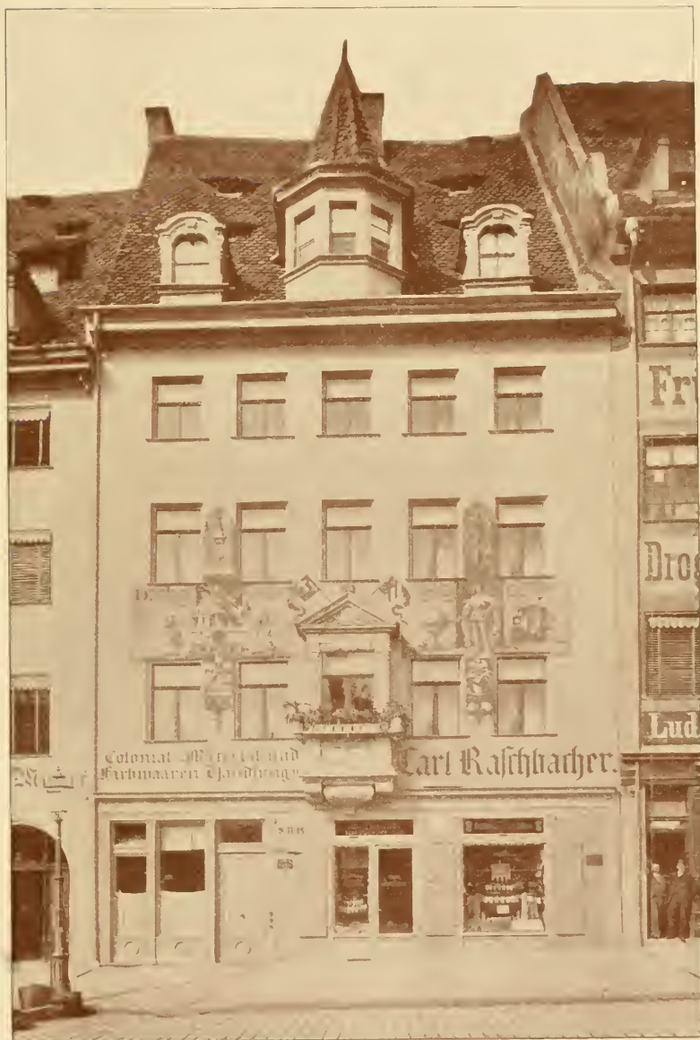
THE "BEHAIM" HOUSE AT NÜRNBERG.
