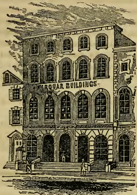
THE FARQUHAR BUILDING.
