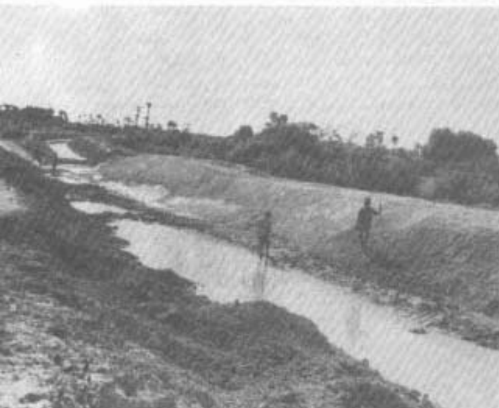
Left: Sodding main irrigation canal to stabilize slopes. Baray, Cambodia. Right: Enlarging main irrigation canal to convey 459 cu. ft. per second. Dragline was furnished by USOM.
