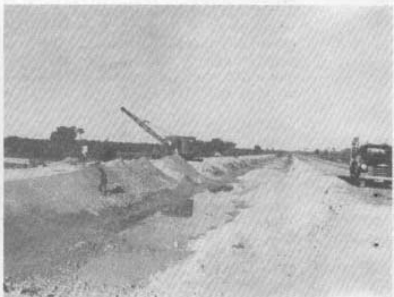
Left: Sodding main irrigation canal to stabilize slopes. Baray, Cambodia. Right: Enlarging main irrigation canal to convey 459 cu. ft. per second. Dragline was furnished by USOM.
