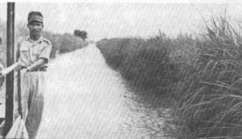
Cambodian canal project for dividing Mekong River flood waters to adjacent croplands for soil improvement. The Mekong carries large amounts of lime from Tibet during flood stage.
