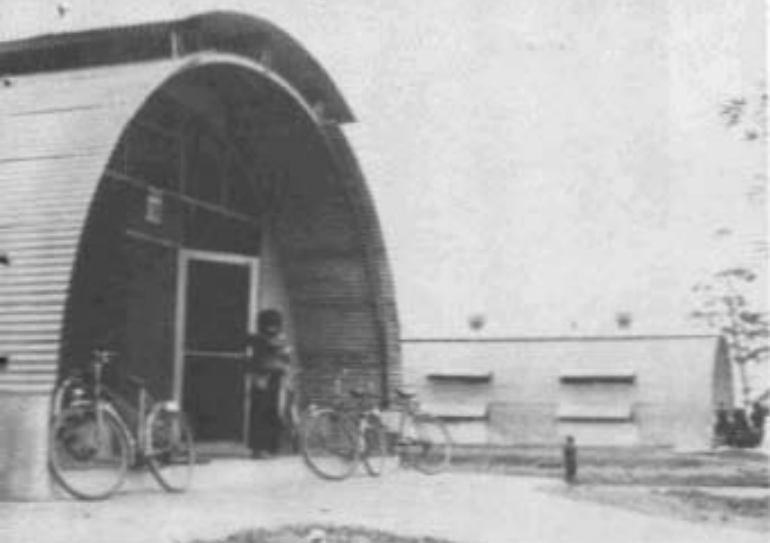
Prefab hospital set up at Sontay.
