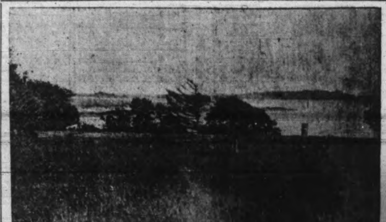
LOOKING SOUTH FROM BLOCK 2.
