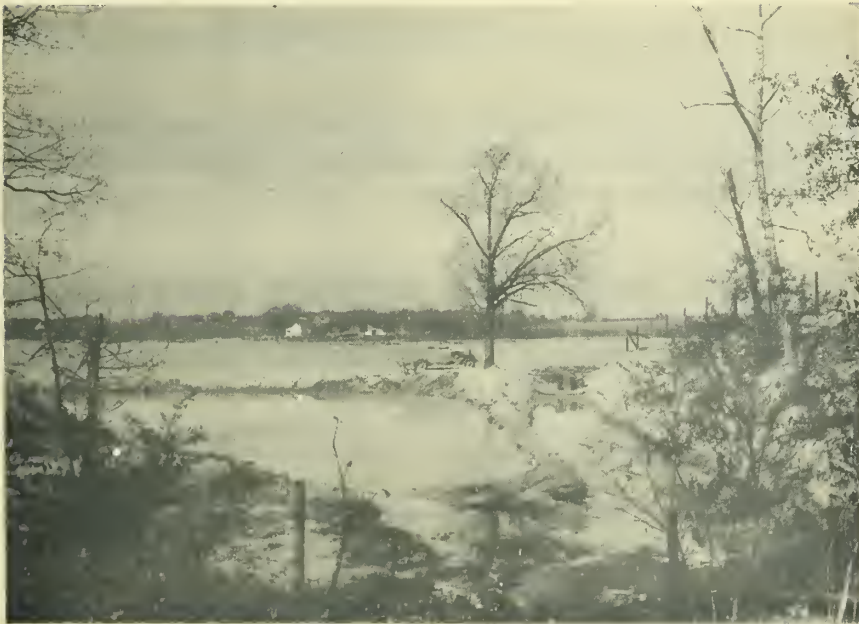
Figure 7.—Silt trap or settling basin behind road fill on east side of Mission Lake.
