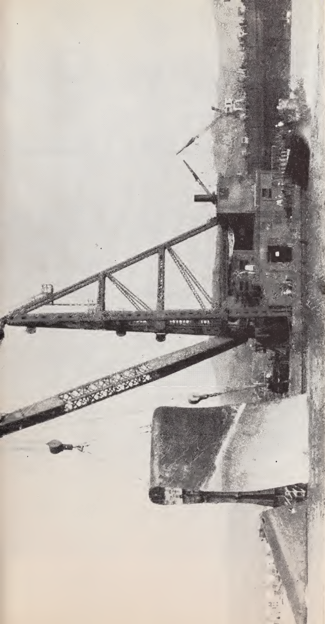
Bow of Pittsburgh—towed in—cut up and restored to the ship.
