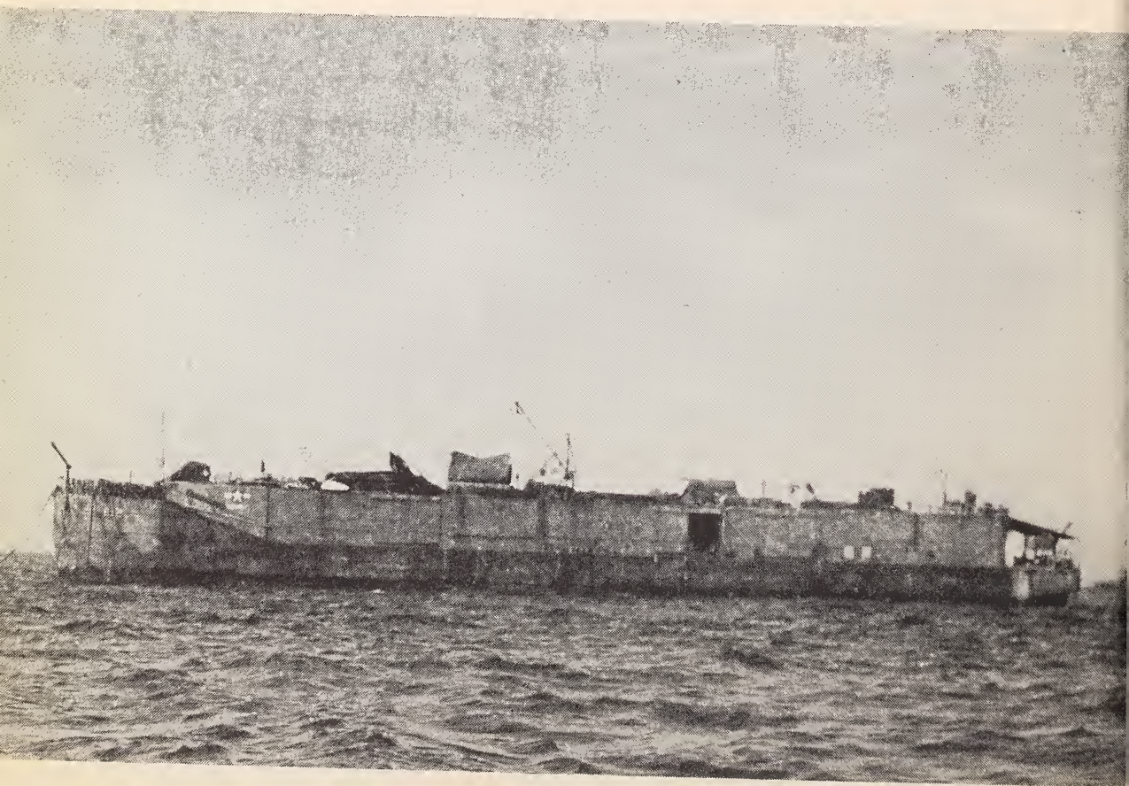
YF Yard Freight Barge (YF-512 stowage and issue of fleet freight)
