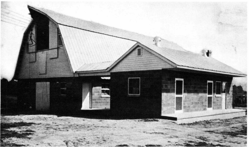
FIGURE 6.—A dairy house consisting of two workrooms and a boiler room, and connected to the barn by a covered passageway.
