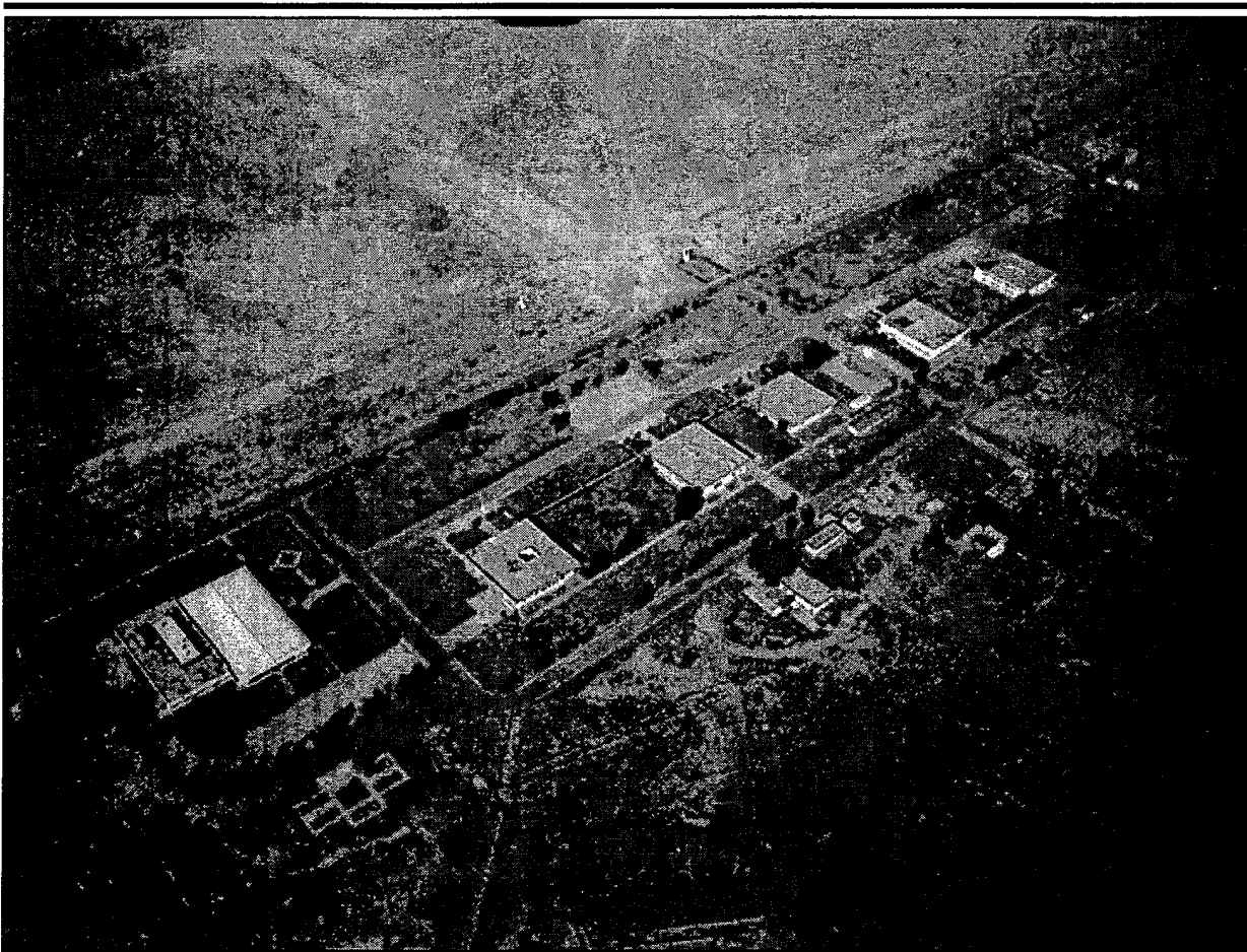
Figure 8. Al Muthanna administration support area razed after 1994.
