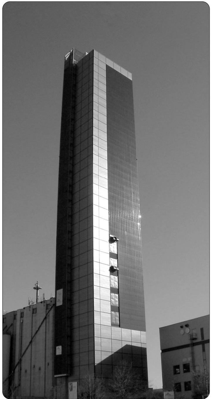
The Schapfen Mill Tower is a flour mill in Germany. The southern facade is faced with 1,300 thin-film solar modules.
