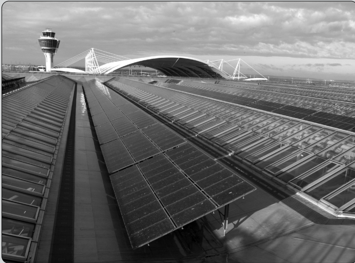
Image courtesy of BP Solar
