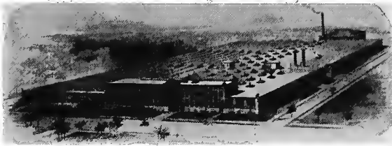
FIG. 25.—Factory of Potter & Johnson Co., Pawtucket, R. I., showing administration front, saw-tooth shop, and power plant, all practically under one roof.
