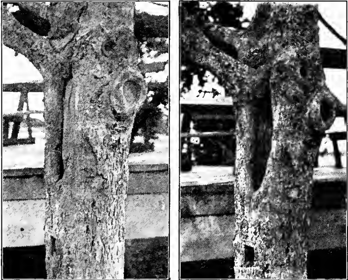
FIG. 153. Decayed tree after and before being filled with concrete.
