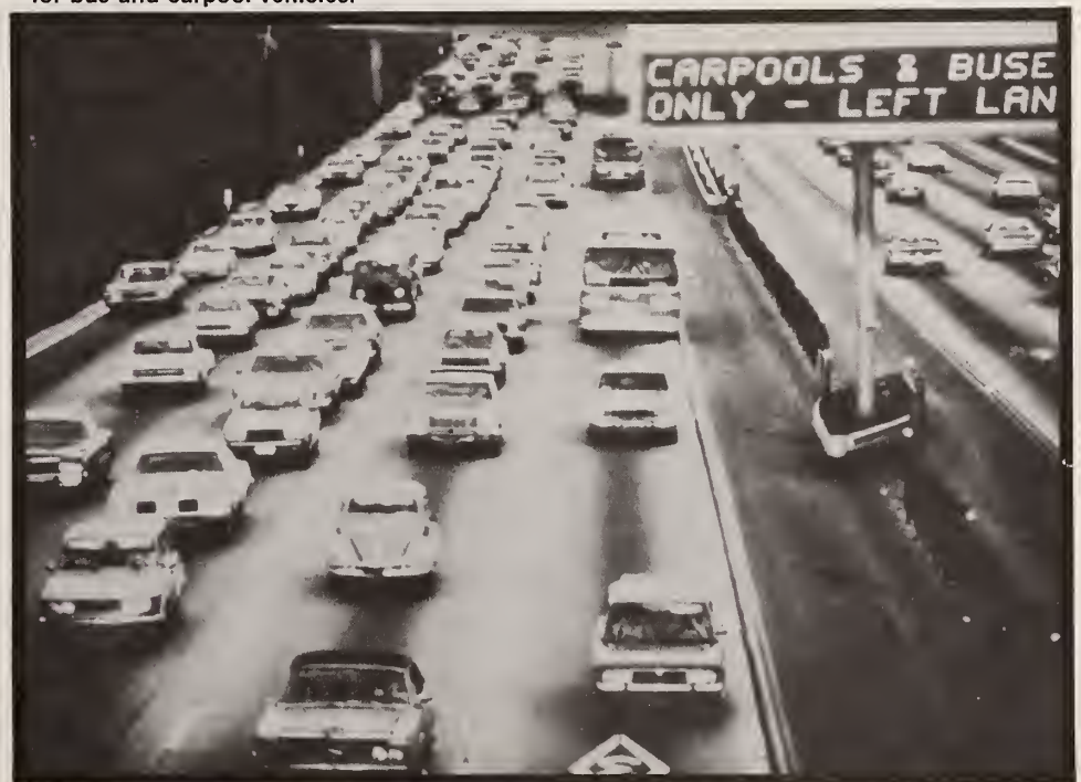
The “diamond lanes” on the Santa Monica Freeway provided concurrent flow reserved lanes for bus and carpool vehicles.
