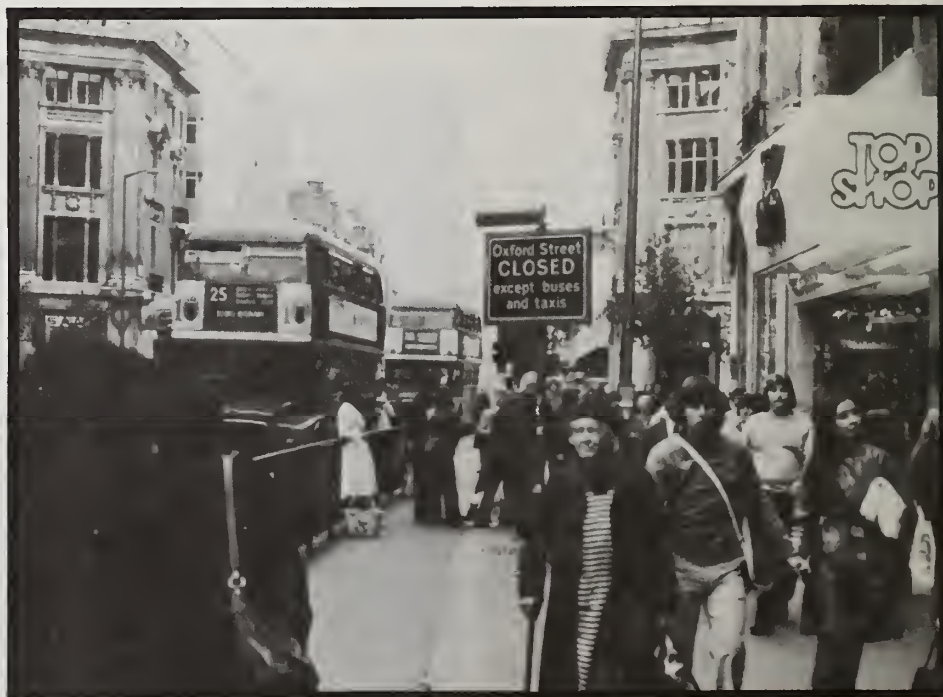
A transit mall on Oxford Street in London, England.
