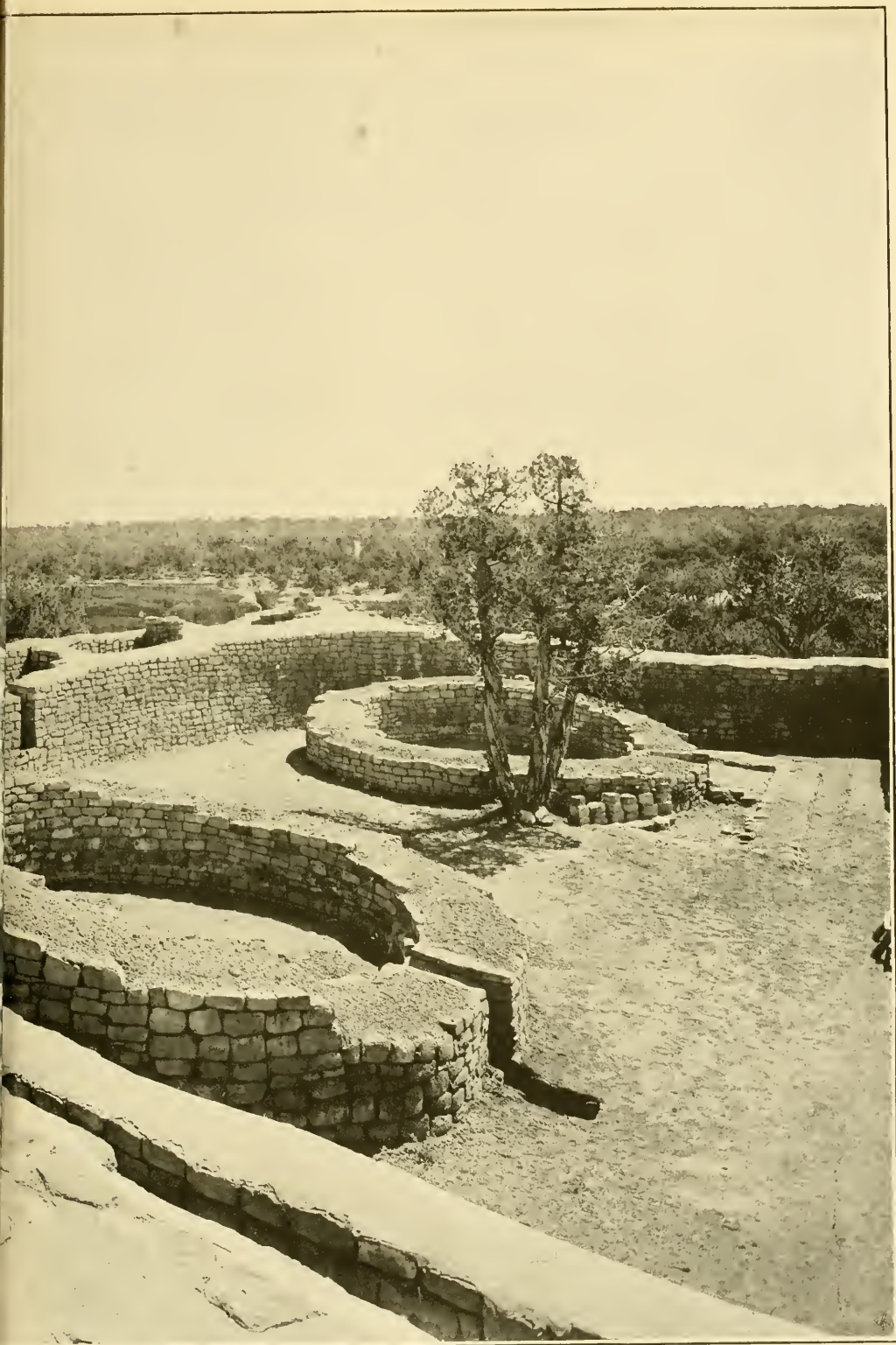
DAR TREE WITH 360 RINGS WHICH WAS CUT DOWN DURING EXCAVATION
