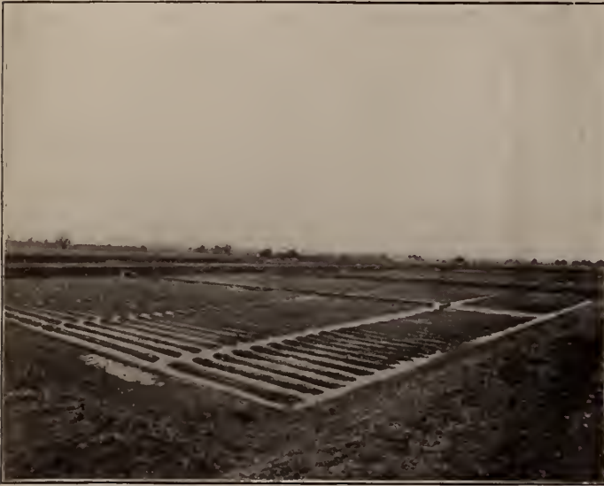
1. Bird's-eye view of sewer beds, showing surface of some of the beds furrowed as they are during the winter months.
