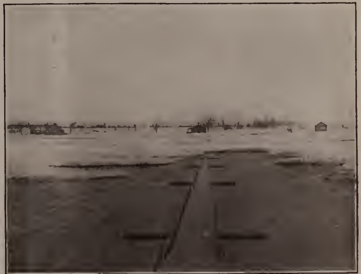
2. Bird's-eye view of the beds, showing the run-way in which the sewage flows to reach the surface of the beds.
