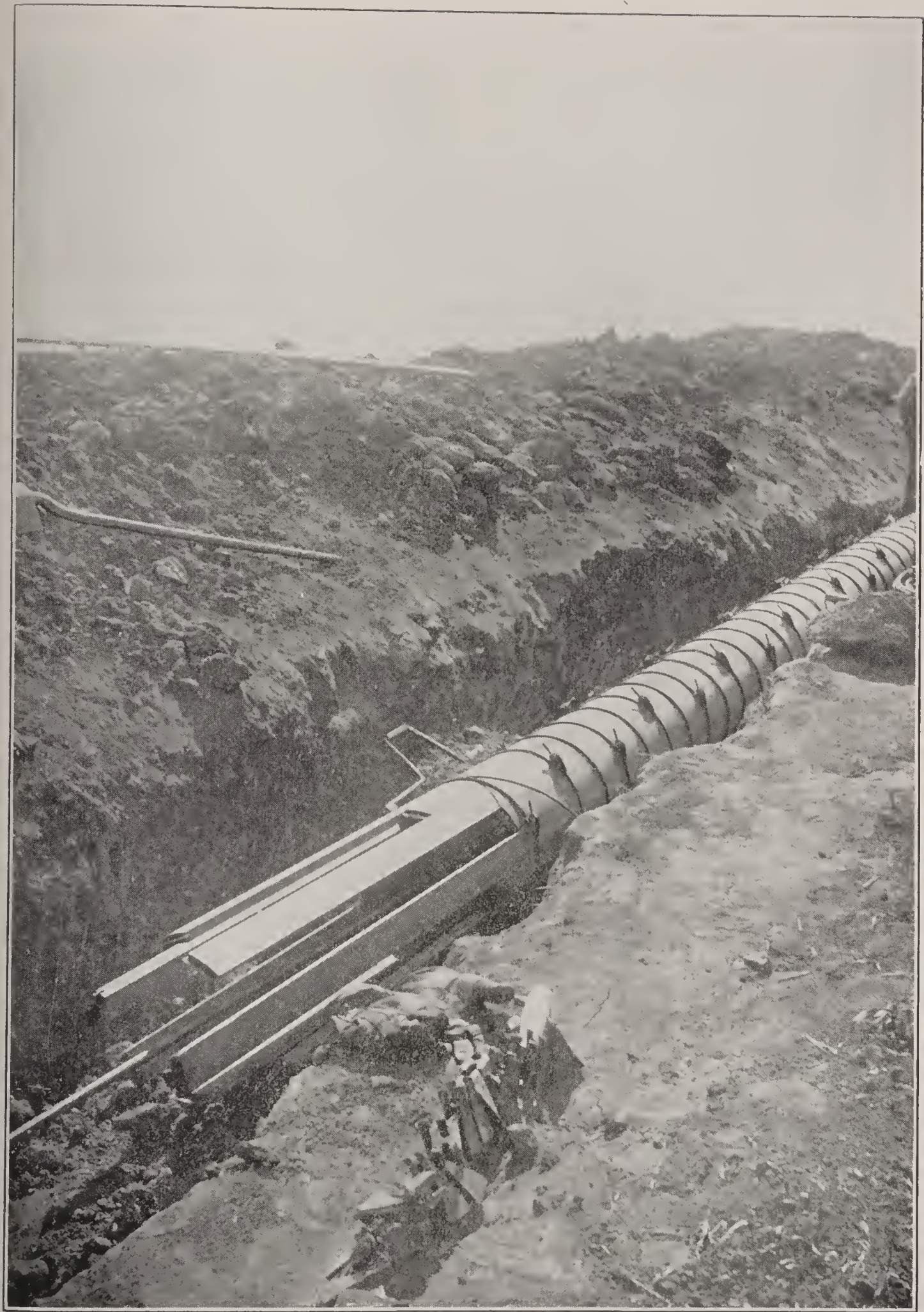
FIG. 147.—WOODEN-STAVE PIPE.
