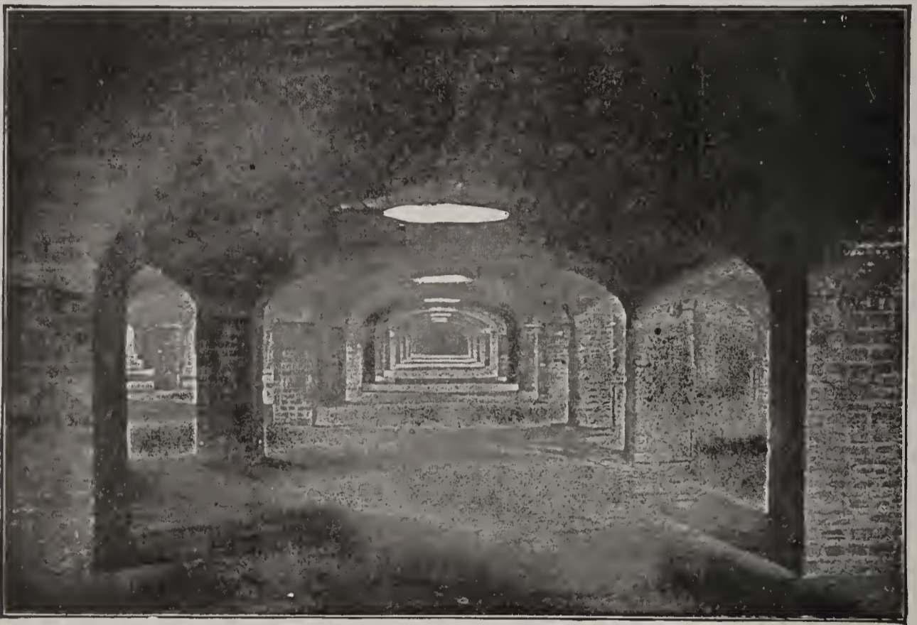
FIG. 122. — INTERIOR VIEW; ALBANY FILTERS. (From Trans. Am. Soc. C. E., vol. XLIII.)
