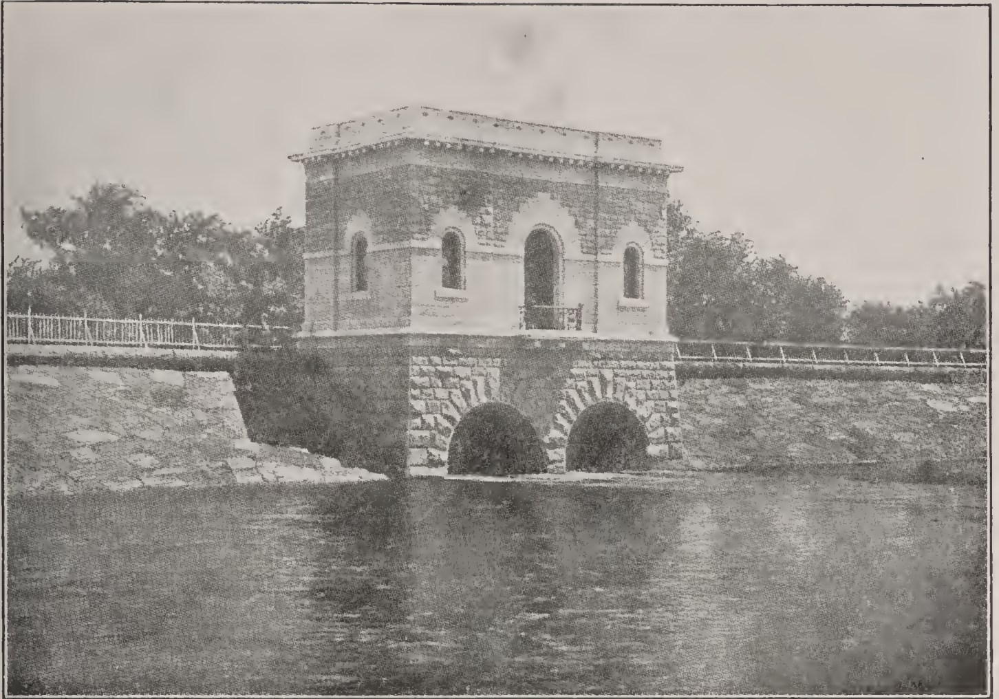
FIG. 84.—CENTRAL PARK GATE-HOUSE, NEW YORK. (WEGMANN.)
