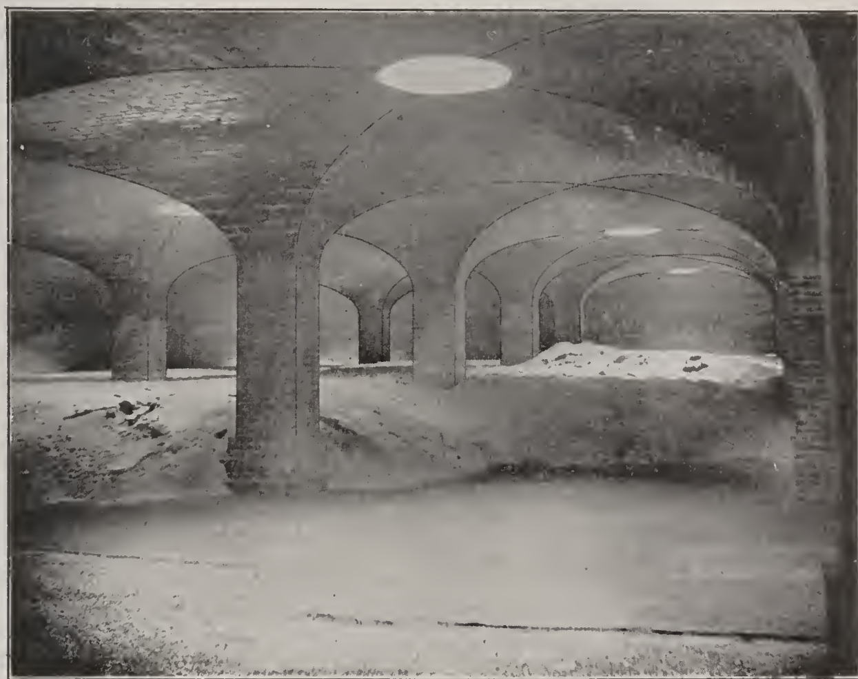
FIG. 201.—COVERED FILTER, ASHLAND, WIS. (From Trans. Am. Soc. C. E., Vol. XLIII.)
