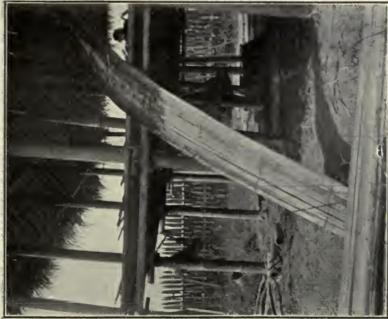
(1) The framework with split bamboo for flooring.
