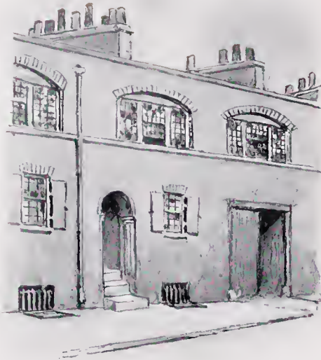
Weavers' Houses, Menotti Street, Bethnal Green. Showing large windows of workshops on top floor.
