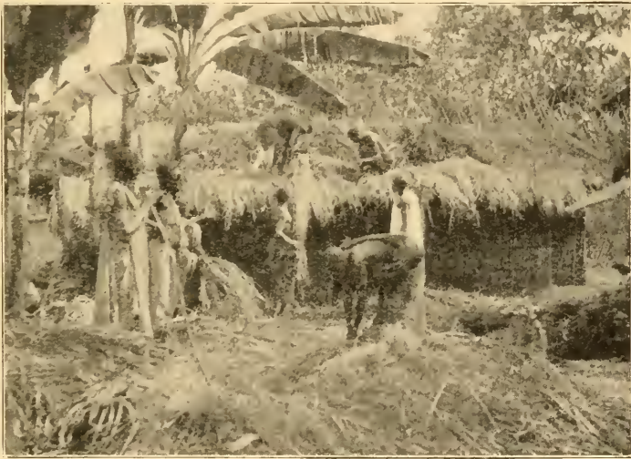
FIG. 60.—THATCHING A HUT.
