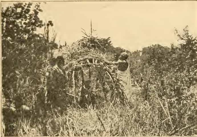
FIG. 55.—BUILDING TEMPORARY HUT.
