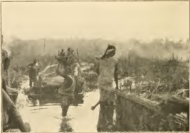
FIG. 36.—MAKING A BRIDGE AND ROAD IN A SWAMP.
