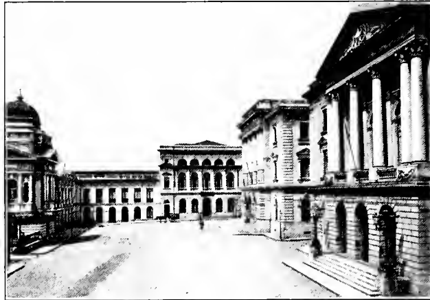
PUBLIC BUILDINGS, SÃO PAULO
