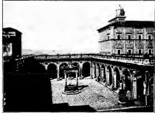
CENTRAL COURT, MONTE CASSINO (Designed by Bramante)
