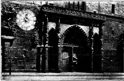
WEST DOOR, CATHEDRAL OF BASLE
