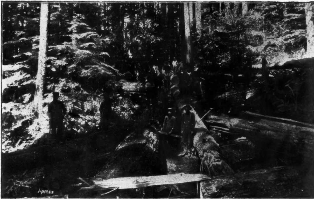
BUILDING TRAMWAY FROM INDEX MINE TO SKYKOMISH RIVER.
