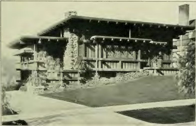
Courtesy of The National Builder .
