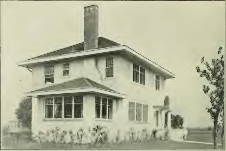
Courtesy of The National Builder .
