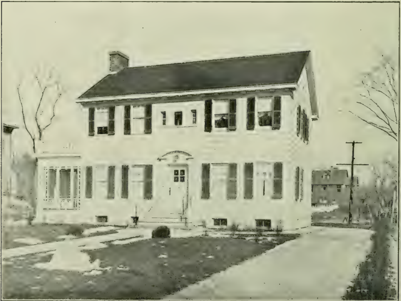
Courtesy of The National Builder .
