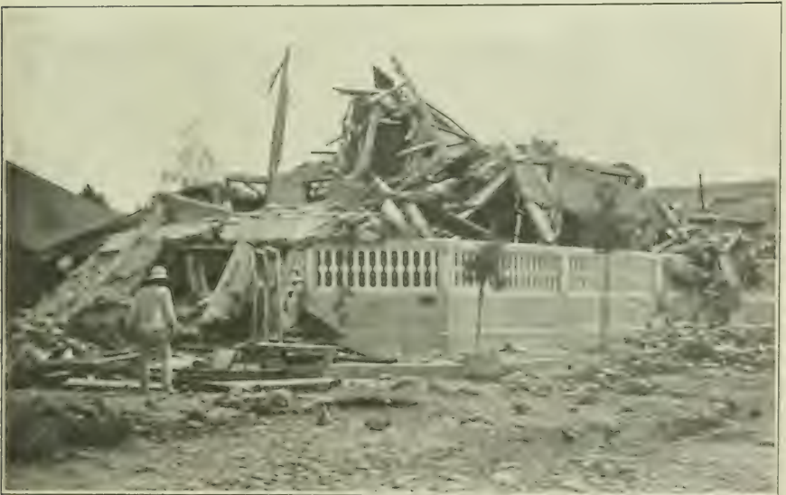
A RUIN OF THE SAN SALVADOR EARTHQUAKE.
