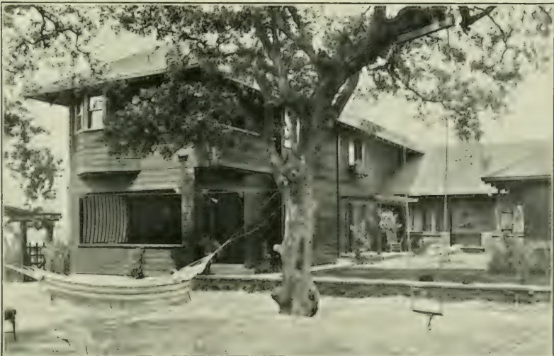
Courtesy of The National Builder .
