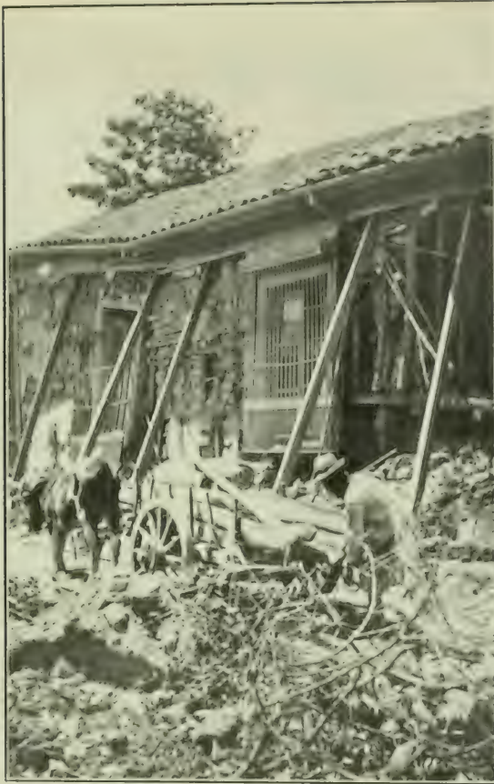
A WRECKED HOUSE IN SAN SALVADOR.
