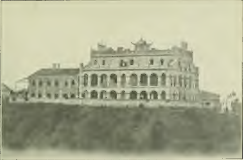
ADMINISTRATION BUILDING, PING HSIANG COLLIERY.
