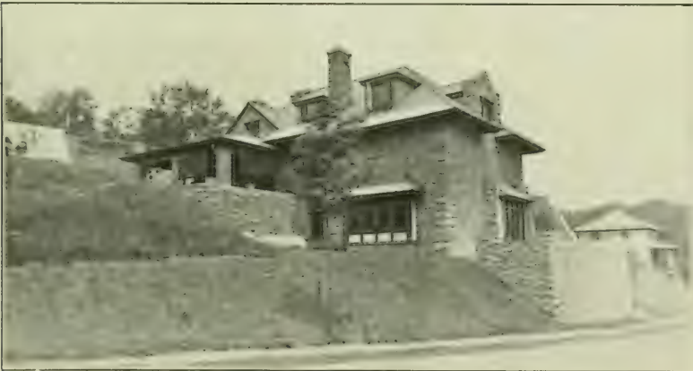
Courtesy of The National Builder .
