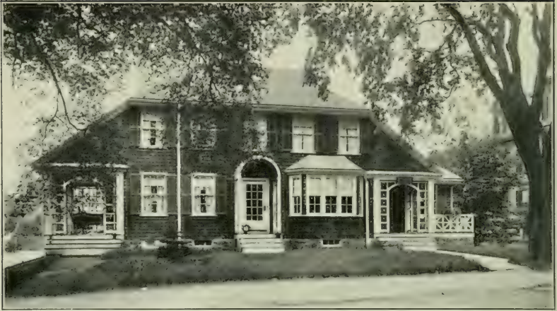
Courtesy of The National Builder .
