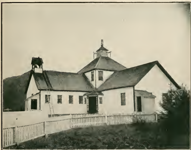
EDUCATIONAL BUILDING AT METLAKAHTLA
