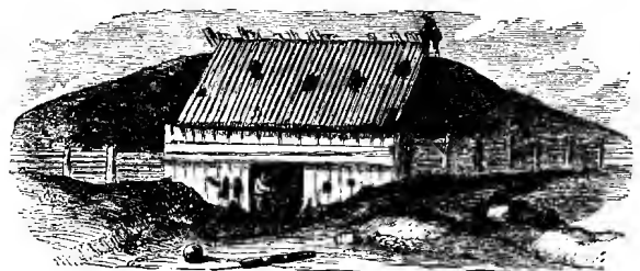
REAR VIEW OF CASEMATE NO. 2.
