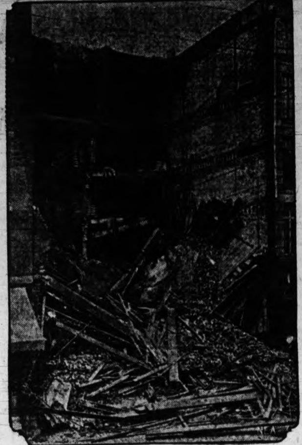
RAIN SENDS BUILDING DOWN—A record-breaking rain-storm in Cincinnati caused the collapse of this building. Four and one-half inches of rain fell in four hours, and the water is believed to have undermined the foundation. The building caved in less than twenty minutes after employees of the Hurlig Bottle Co., which occupied it, had left.
