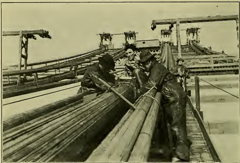
"SEVERAL STRANDS WERE SQUEEZED TOGETHER ---- TO FORM A CORE."— See page 107.
