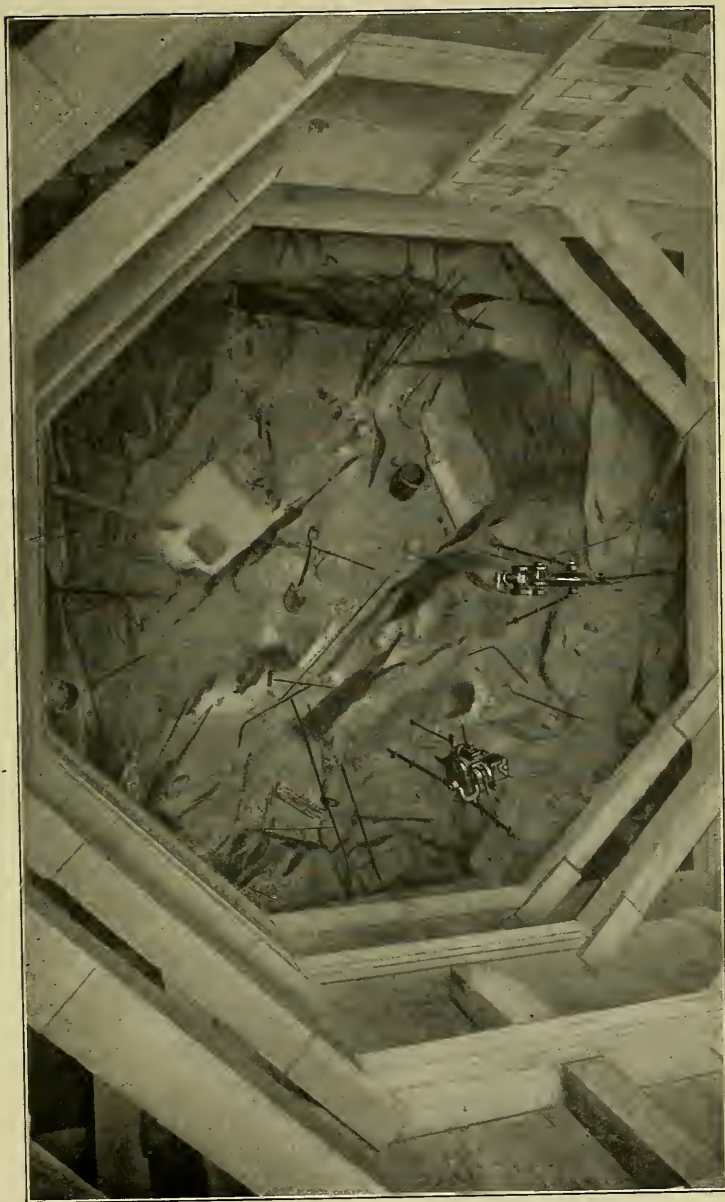
DRIVING AN AQUEDUCT SHAFT. NOTE THE PNEUMATIC DRILLS MOUNTED ON TRIPODS.
