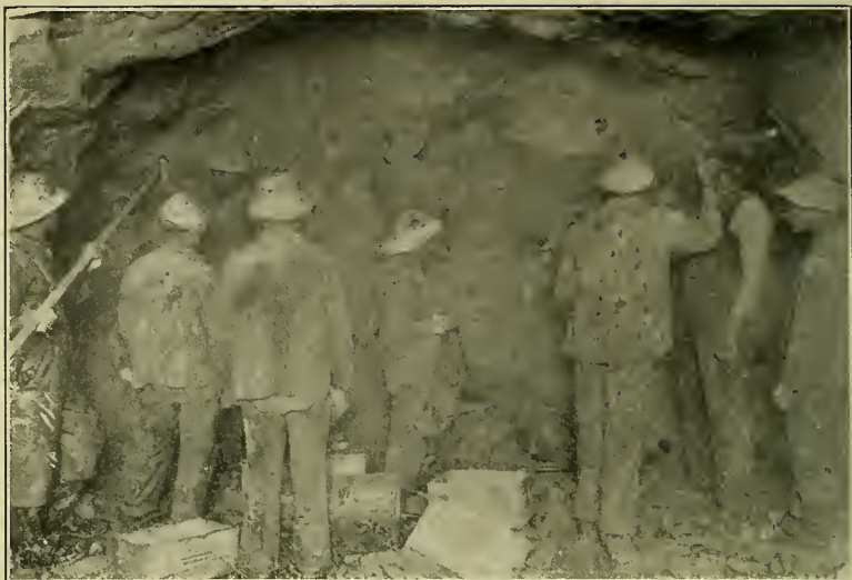
RAMMING THE POWDER INTO THE SHOT HOLES.
