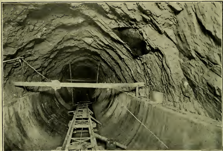
SECTION OF THE TUNNEL WITH SIDE WALLS CONCRETED.
