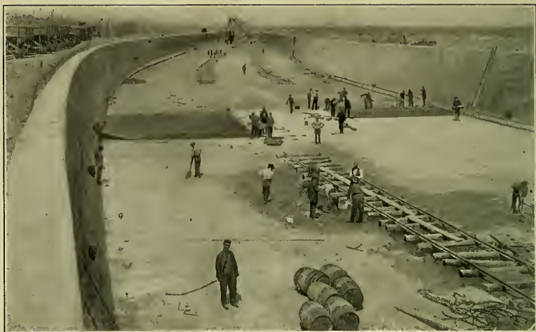
WATERPROOFING A TROUGH AT IRONDEQUOIT CREEK CROSSING OF THE AQUEDUCT.
