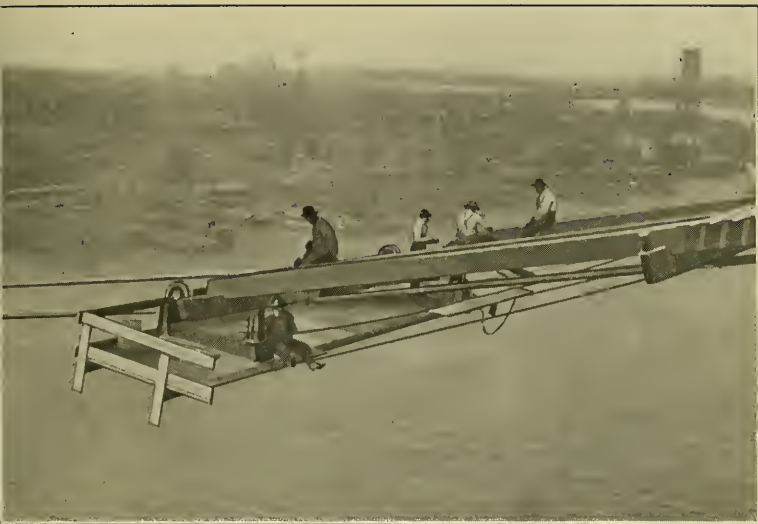
BUILDING A TEMPORARY FOOT BRIDGE ACROSS THE RIVER.
