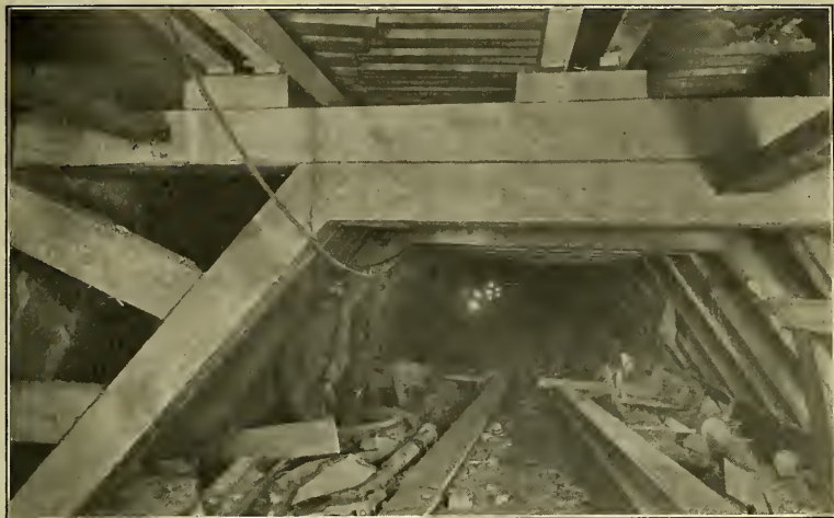
A ROOF OF STEEL WHERE THE ROCK IS SHAKY.
