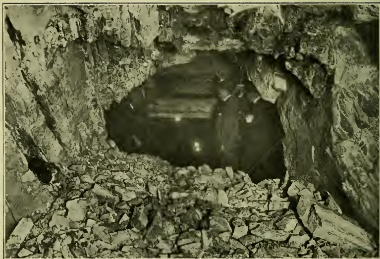
"HOLED THROUGH" FROM ONE SHAFT TO ANOTHER.
