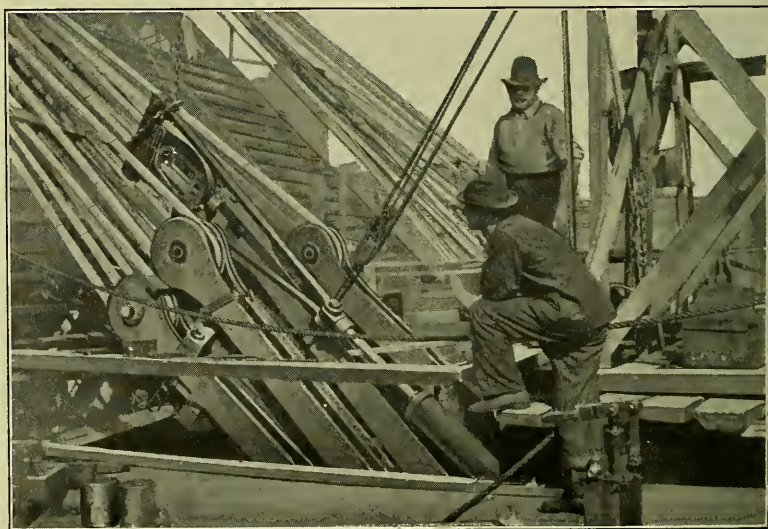
TURNING THE SHOE ON EDGE AND FITTING IT BETWEEN THE EYE BARS.
