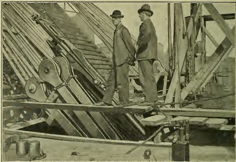
DRAWING BACK THE SHOE WITH A HYDRAULIC JACK.
