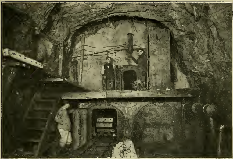
CONCRETE BULKHEAD WITH THREE AIR-LOCKS.
