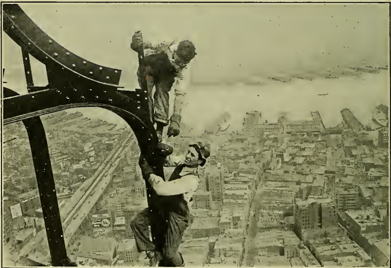
HAND RIVETING WHERE PNEUMATIC HAMMERS CANNOT BE USED.
