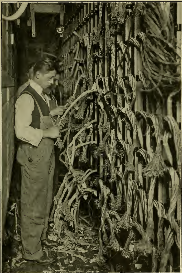
CONNECTING UP A TANGLE OF WIRES BACK OF THE RELAY BOARD.
