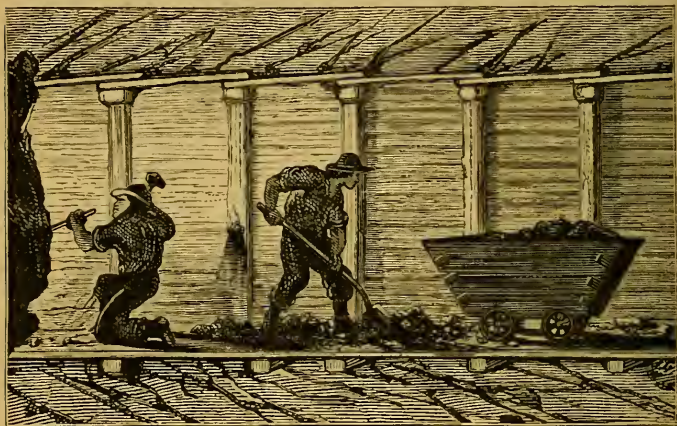
Longitudinal View of Timbered Level.
