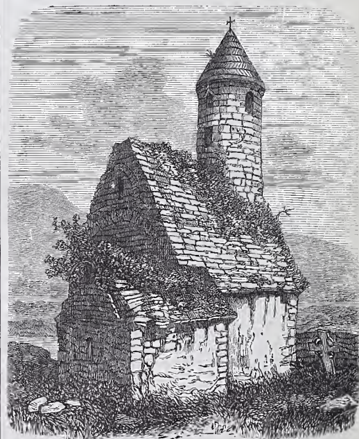
Fig. 2207. St. Kevin's „Küche“ in Glendalough.
